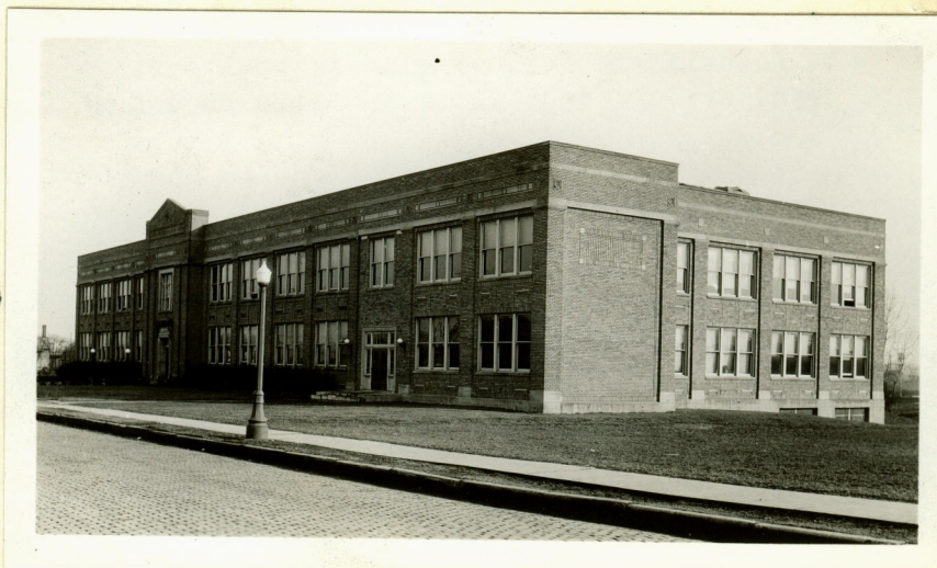
NORTH WEST VIEW
