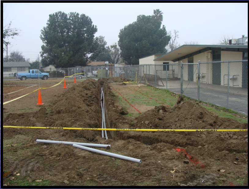
Fairview Elementary - Replacement of underground wiring to Bldg 2
