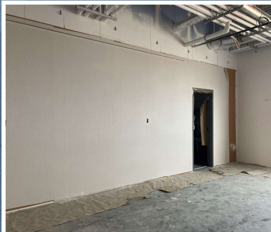
Vinyl Wall Coverings Ongoing
