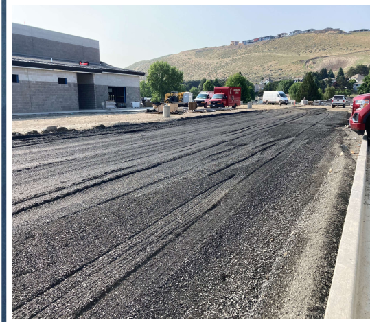
Bus Drop Off Crushed Rock
