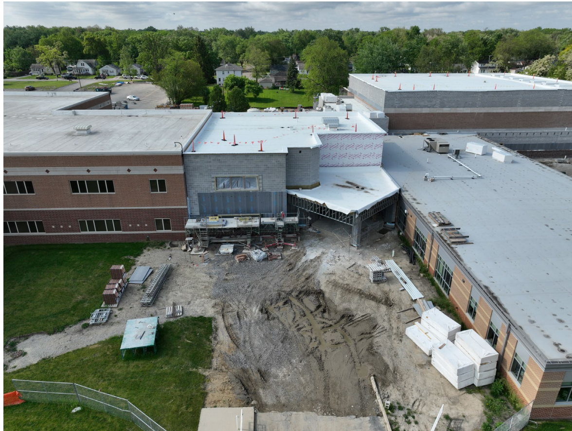
Classroom Addition Exterior
