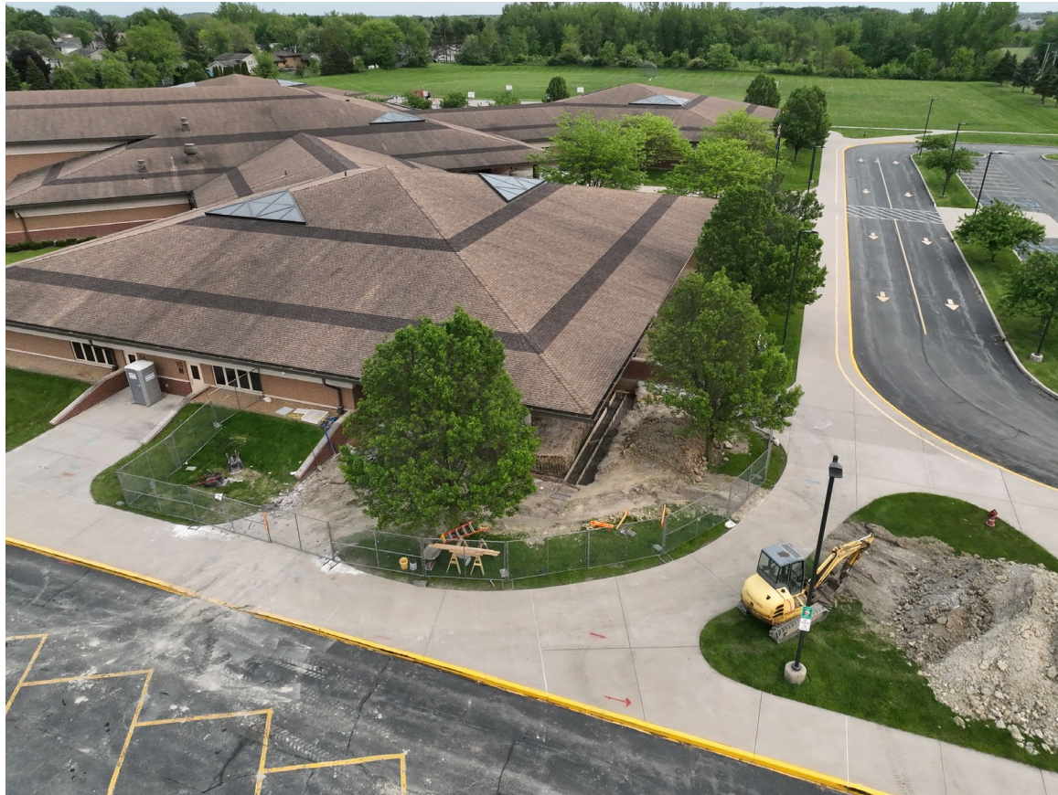
Ariel View of Site Work
