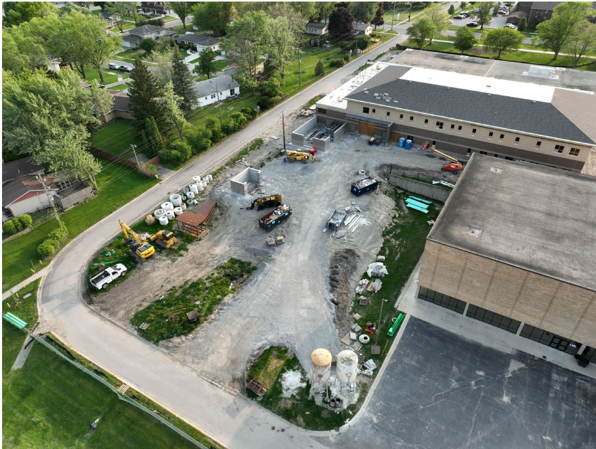
New Administration Side View
