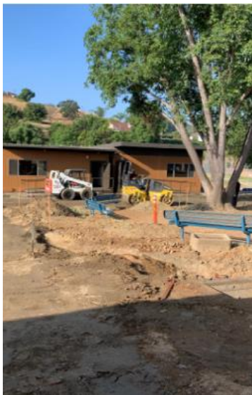
GRADING FOR PAVING
