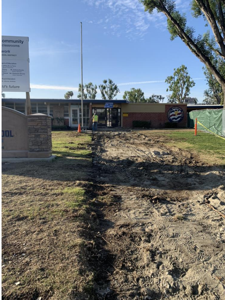
Before ADA Path of Travel Improvements
