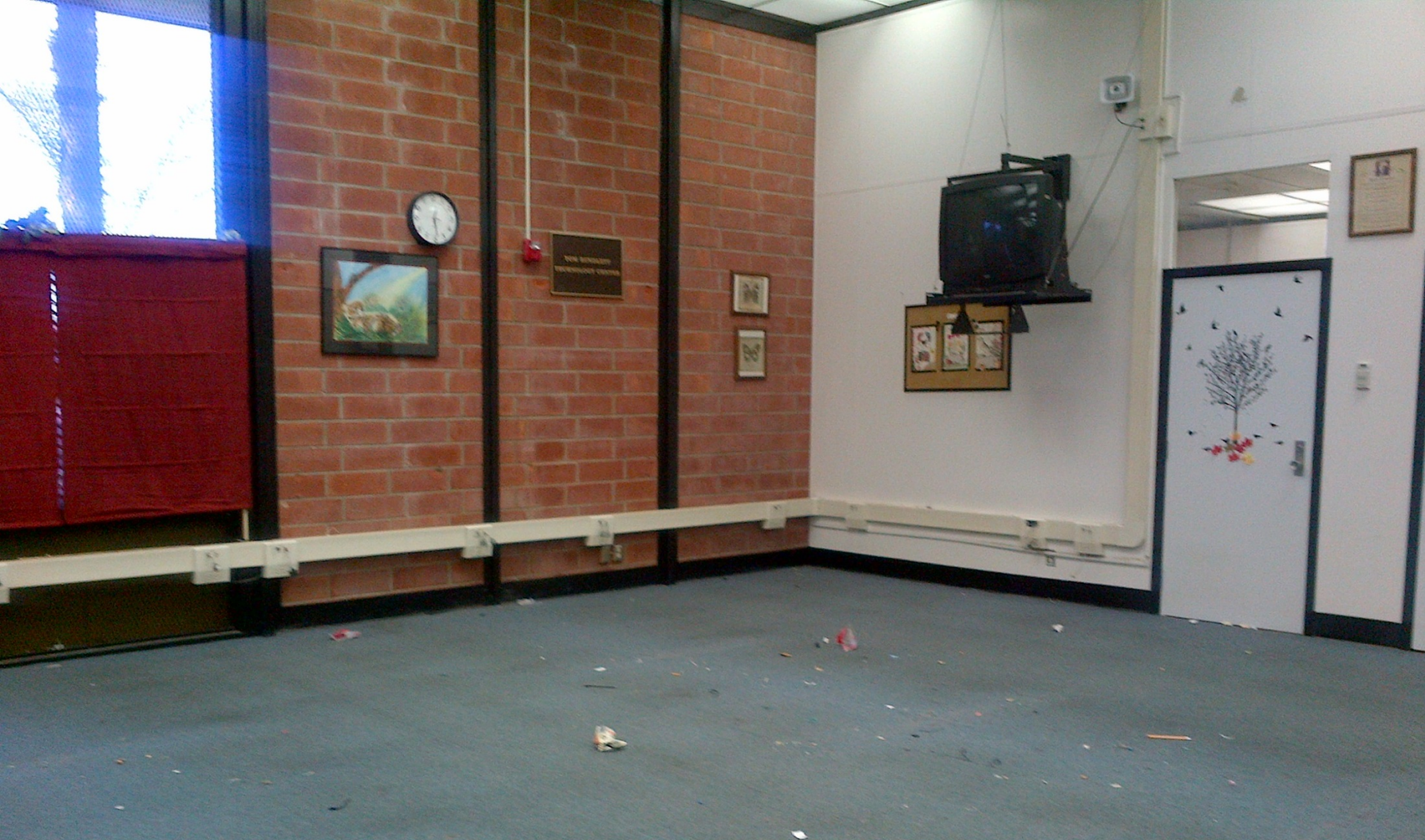
Building the First Three CCCS Technology Labs: Day 1 – Wilson Media Center Before... NCS technicians and Facilities staff worked together to clear out the old computers and furniture from the Wilson High School media center. In this photo, the media center is cleared out and ready to accept the new computers and furniture.
