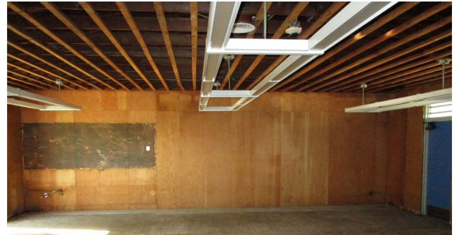
After demolition of wall, floor, and ceiling
