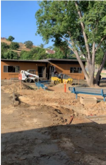
GRADING FOR PAVING
