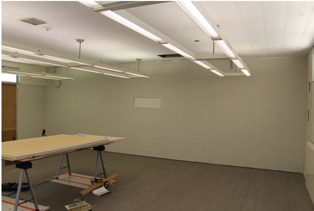
WALL & FLOOR FINISHES
