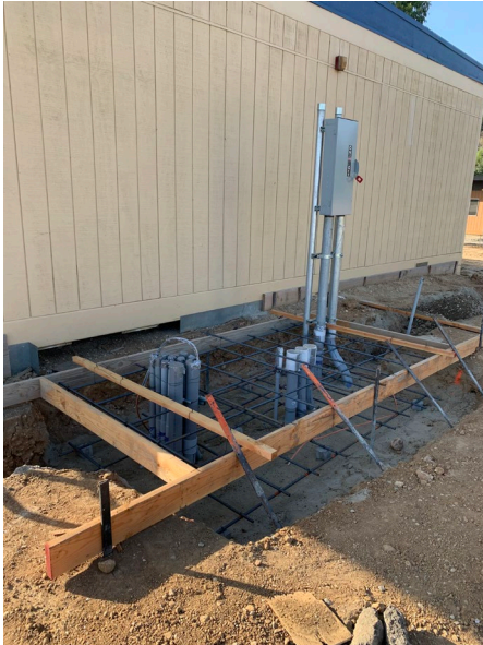
UTILITY PAD FORMS
