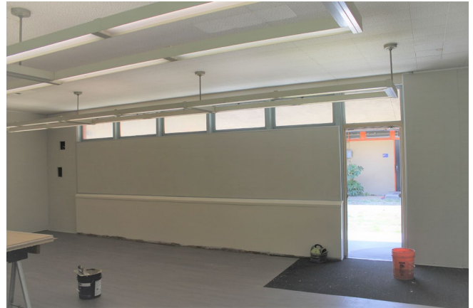
WALL & FLOOR FINISHES
