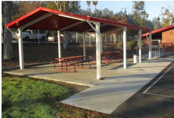
Wing Lane – Concrete for Shade Structure
