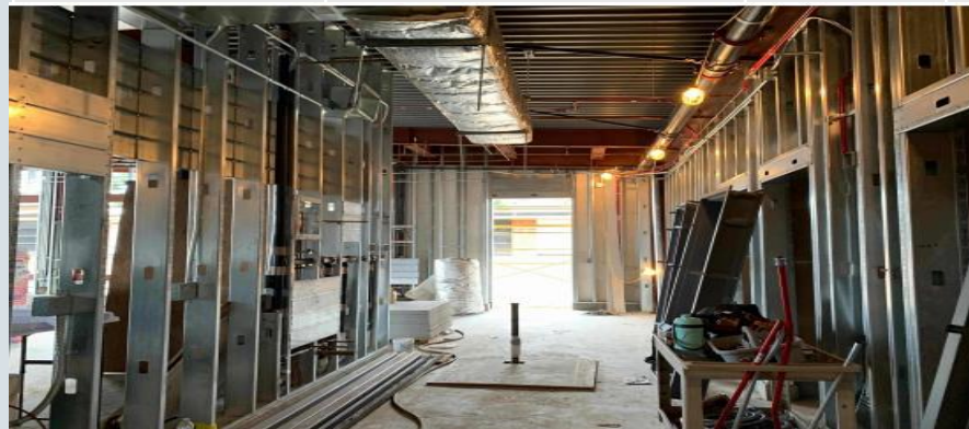
La Puente HS Kitchen: New Kitchen Hallway, Arrival of Door Frames & Finished Metal Framing, Drywall, Insulation Installed
