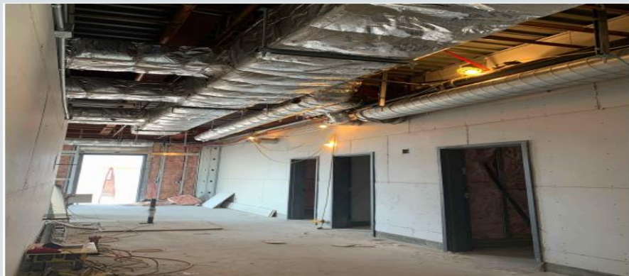
La Puente HS Kitchen: New Kitchen Hallway, Arrival of Door Frames & Finished Metal Framing, Drywall, Insulation Installed
