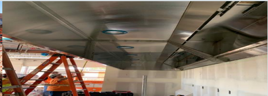
La Puente HS Kitchen – Installing the Kitchen Hood and countertops
