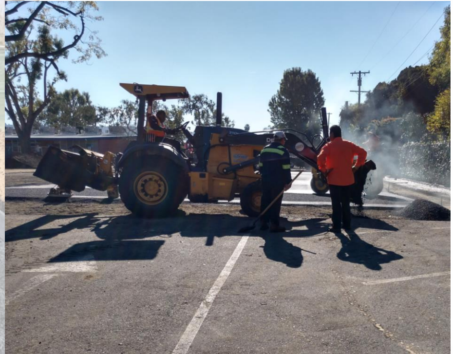
Building Pads North Parking Lot
