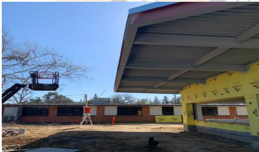
La Puente HS Kitchen – Metal Deck is Being Spray Painted
