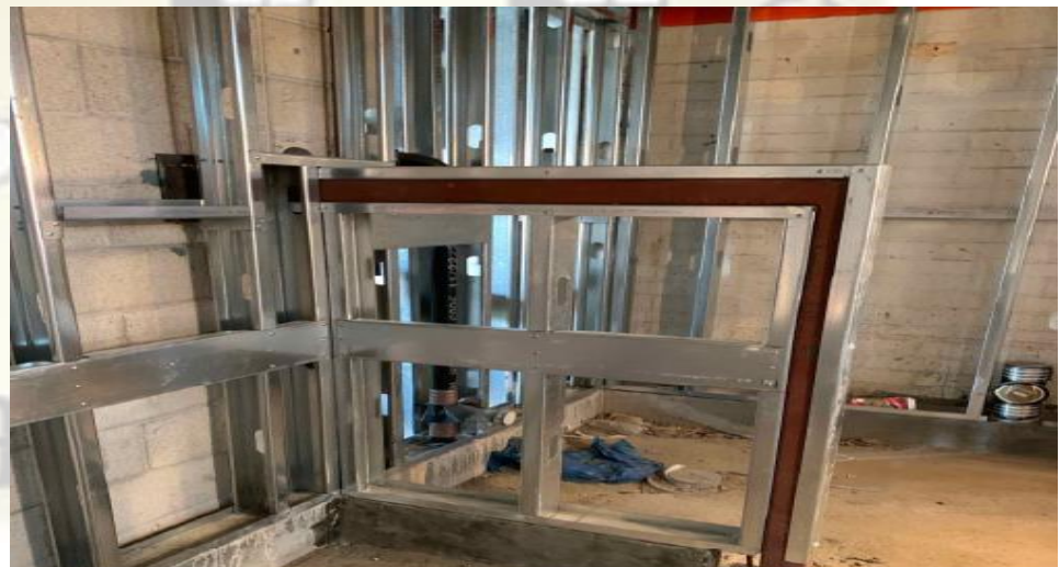
La Puente HS Pool – Structural Pony Wall Completed
