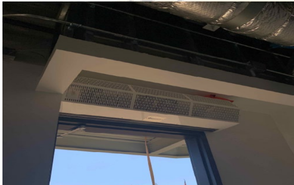
La Puente HS Kitchen – Aircurtain Installed
