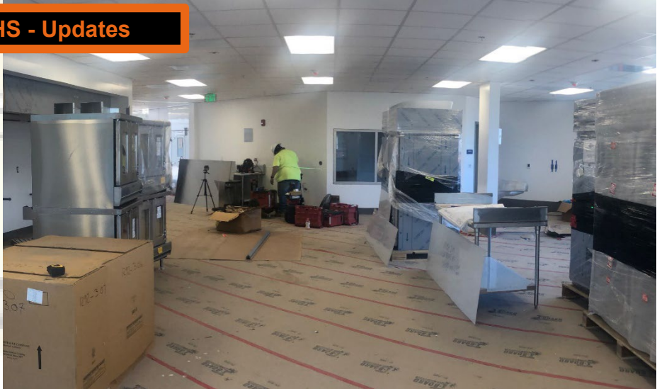
Kitchen – Equipment being installed
