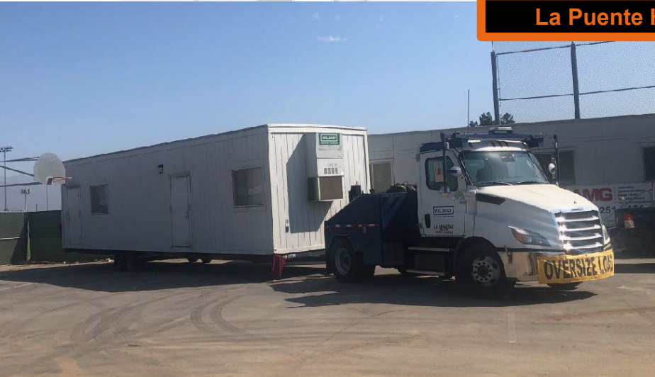
Contractors removing construction trailers
