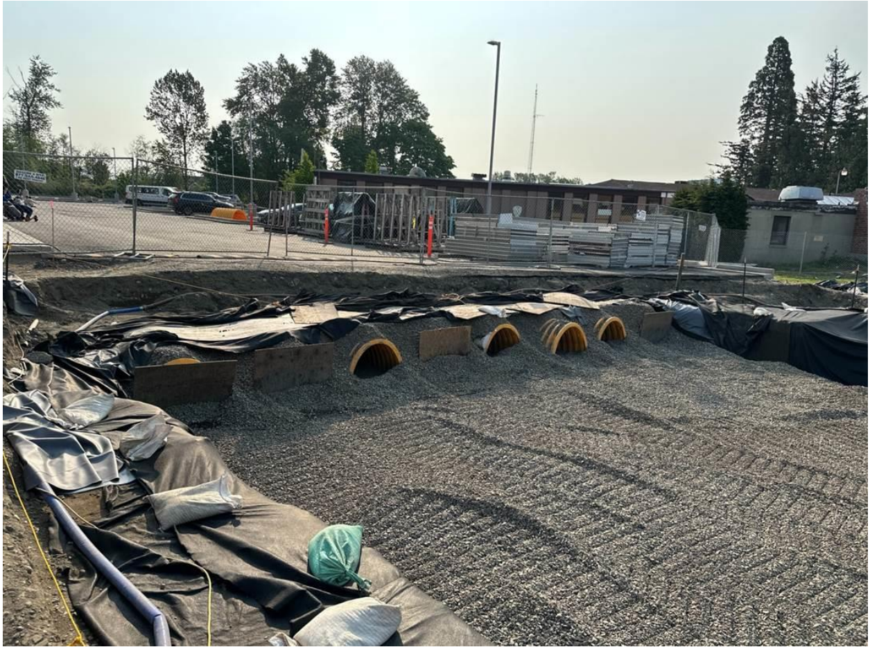
The final underground stormwater detention system was installed this week
