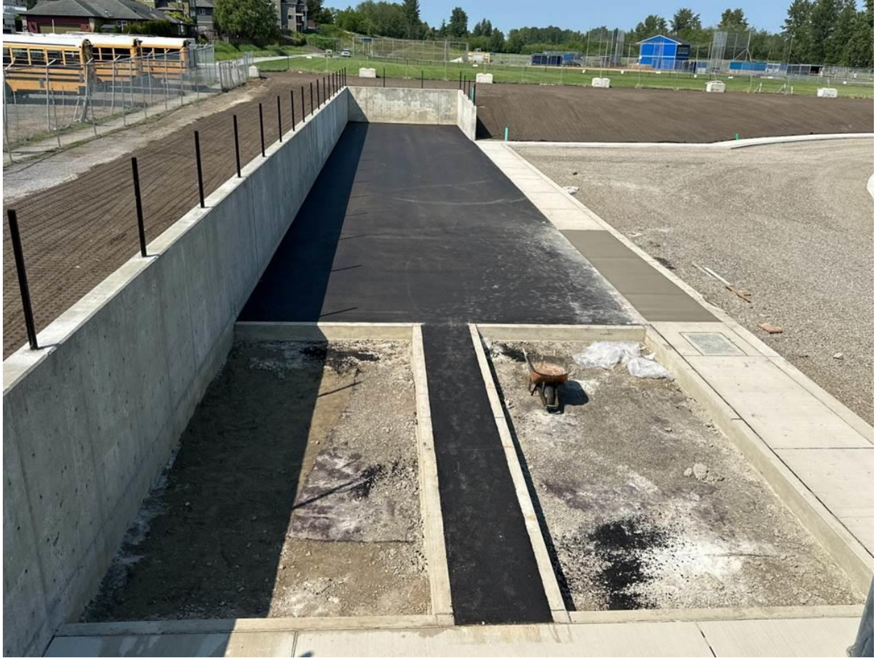
The running surface base in the long jump area
