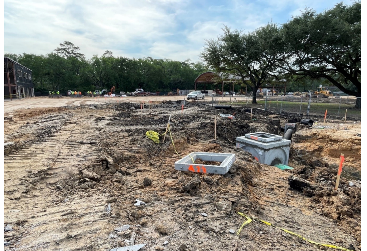
Underground storm water installation with gym and former library in the background
