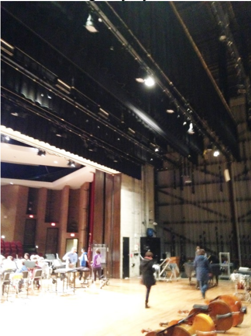
Overhead Stage Fly System
