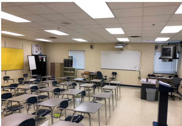
LIGHT FIXTURES IN CLASSROOMS
