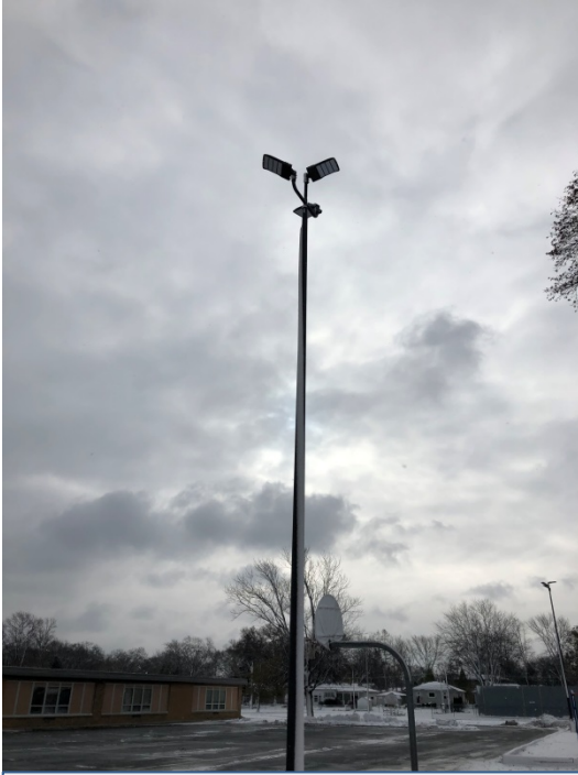
PARKING LOTS HAVE LED LIGHTING
