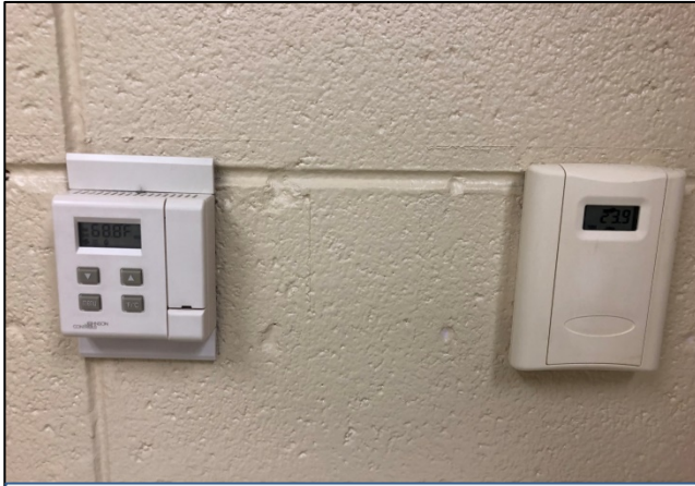
DIGITAL CONTROL SENSORS
