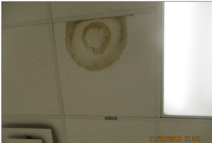
FAN COIL UNITS AND VAV BOXES ARE INSTALLED ABOVE THE CEILING
