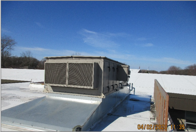
TYPICAL ROOF MOUNTED AIR HANDLING UNIT
