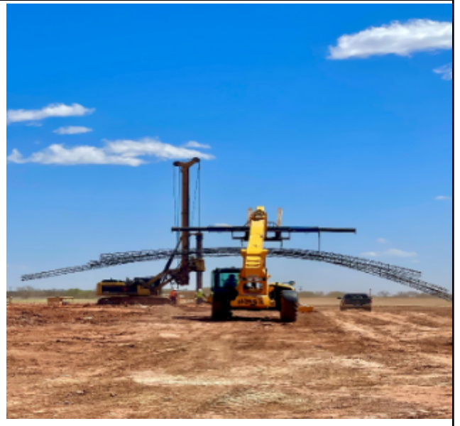
Pier Drilling
