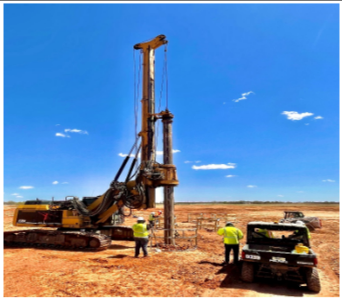
Pier Drilling
