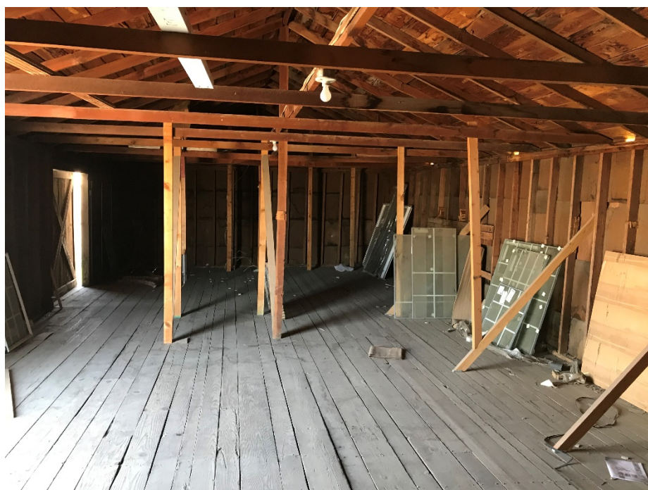
Photo 6. Building #3, view of west interior of building.
