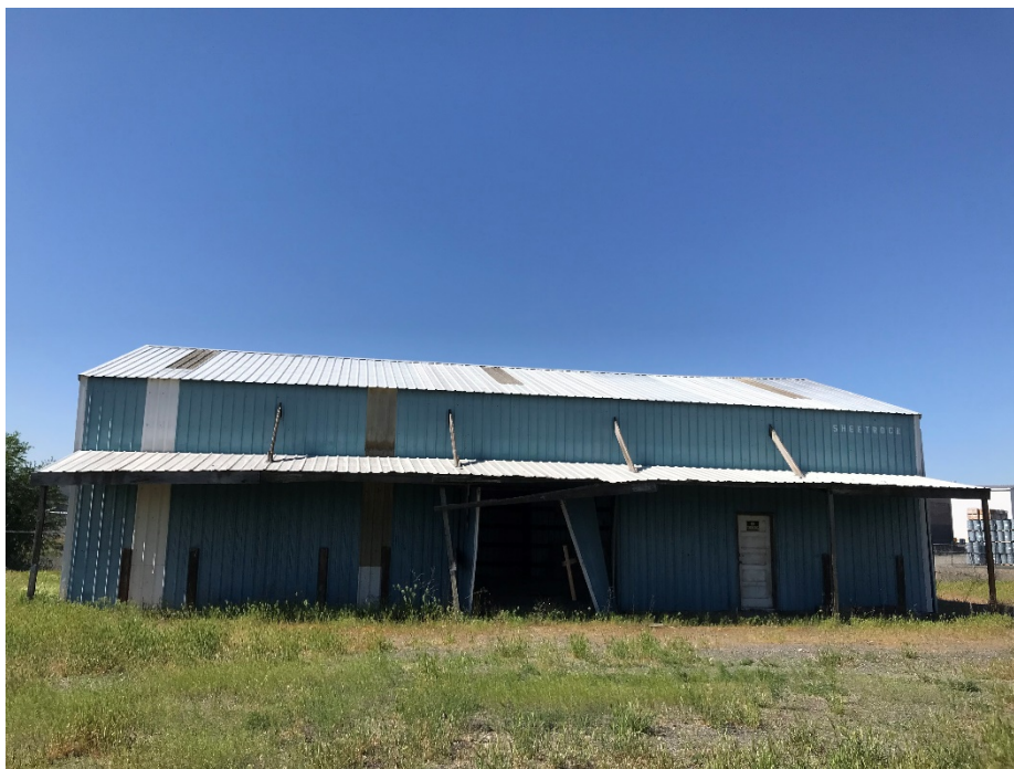
Photo 1. Building #1, view from north of building.
