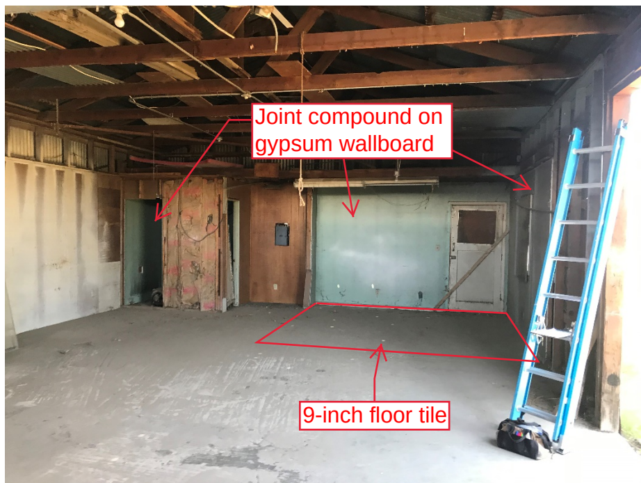
Photo 12. Building #5, view of north interior showing gypsum wallboard with asbestos-containing joint compound and area of asbestos-containing 9-inch vinyl floor tile.
