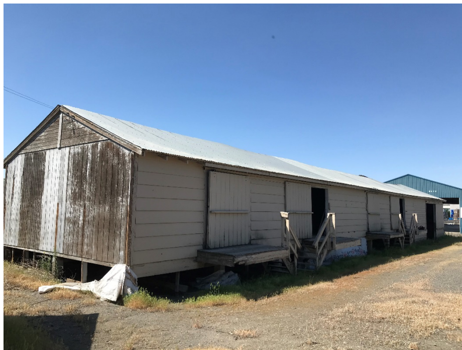
Photo 5. Building #3, view from northeast side of building.
