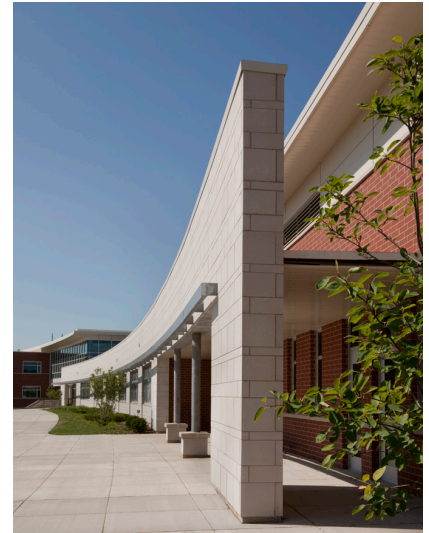
Hubble Middle School 2010 Midwest Construction Project of the Year
