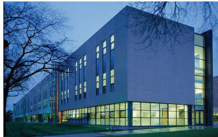
Niles North and West High Schools are the first high schools in Illinois to register for LEED EB: O&M (Existing Building: Operations and Maintenance). This assessment details the physical and operational system modifications required to certify these schools.
