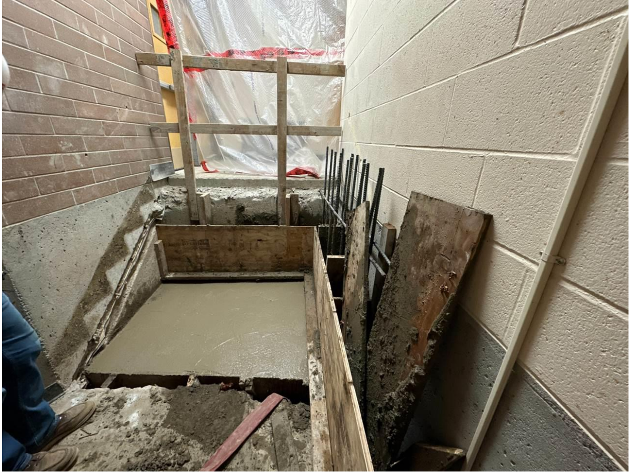
Footings for the new shear walls in the Performing Arts Center
