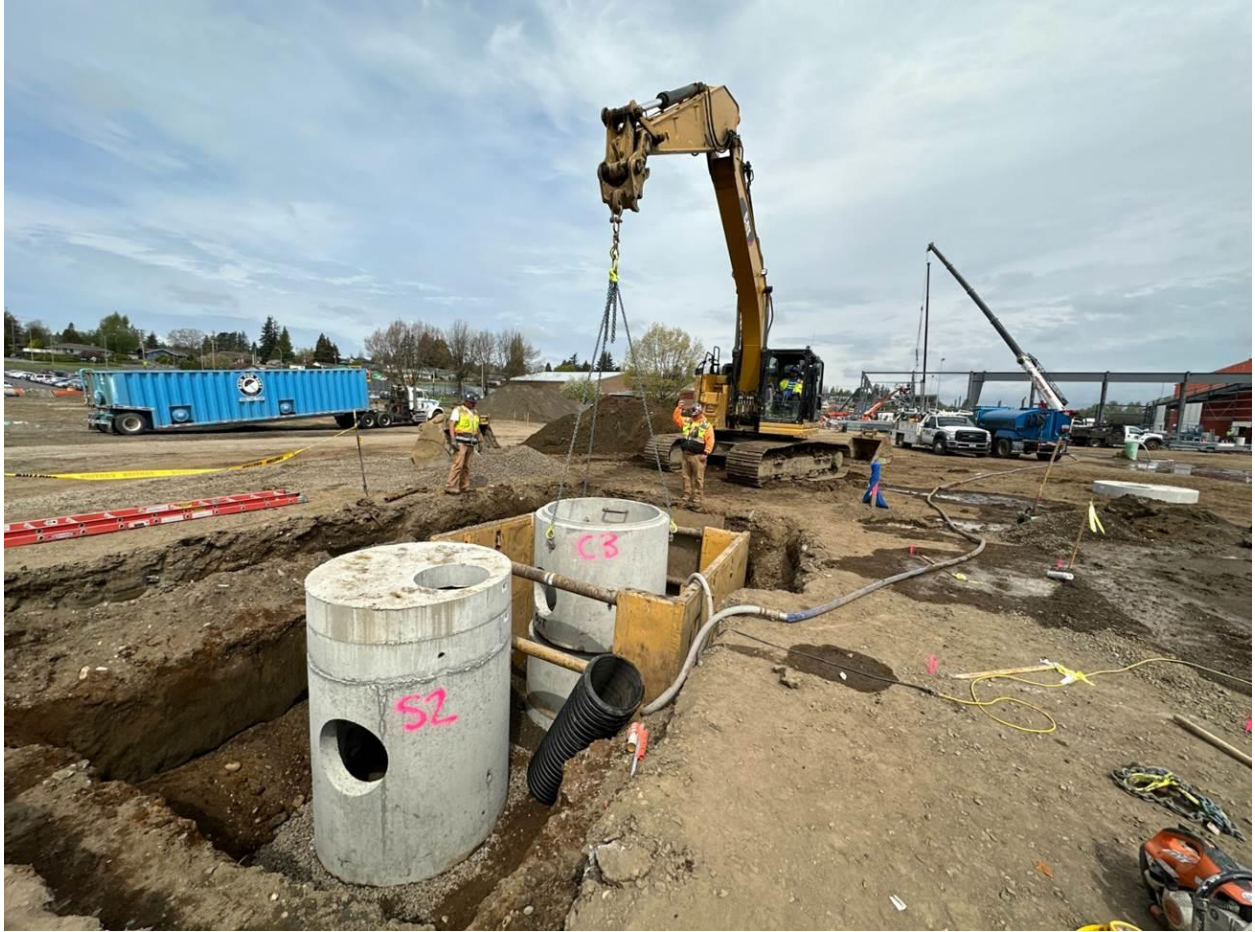
Concrete structures being installed for the underground stormwater system
