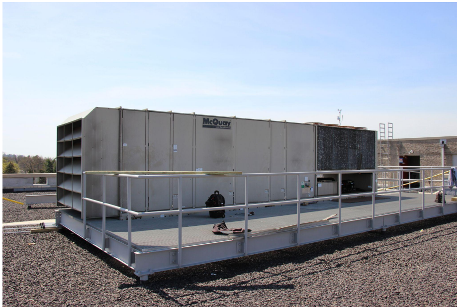
MS Rooftop Heating/Cooling Units
