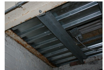
Photo #13 Rusted Steel Roof Over Mechanical Room Stair
