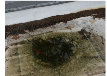
Photo #12 Clogged Roof Drain
