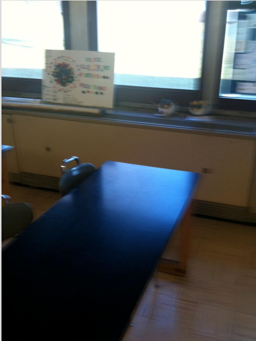
Unit Vent/No Wall Insulation
