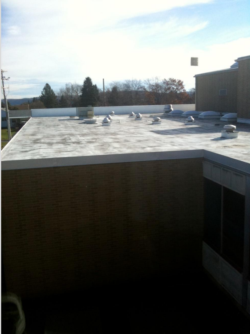
Typical Roof Area-Installed in 1988 (rubber roof) Recoated to extend life cycle of rubber membrane
