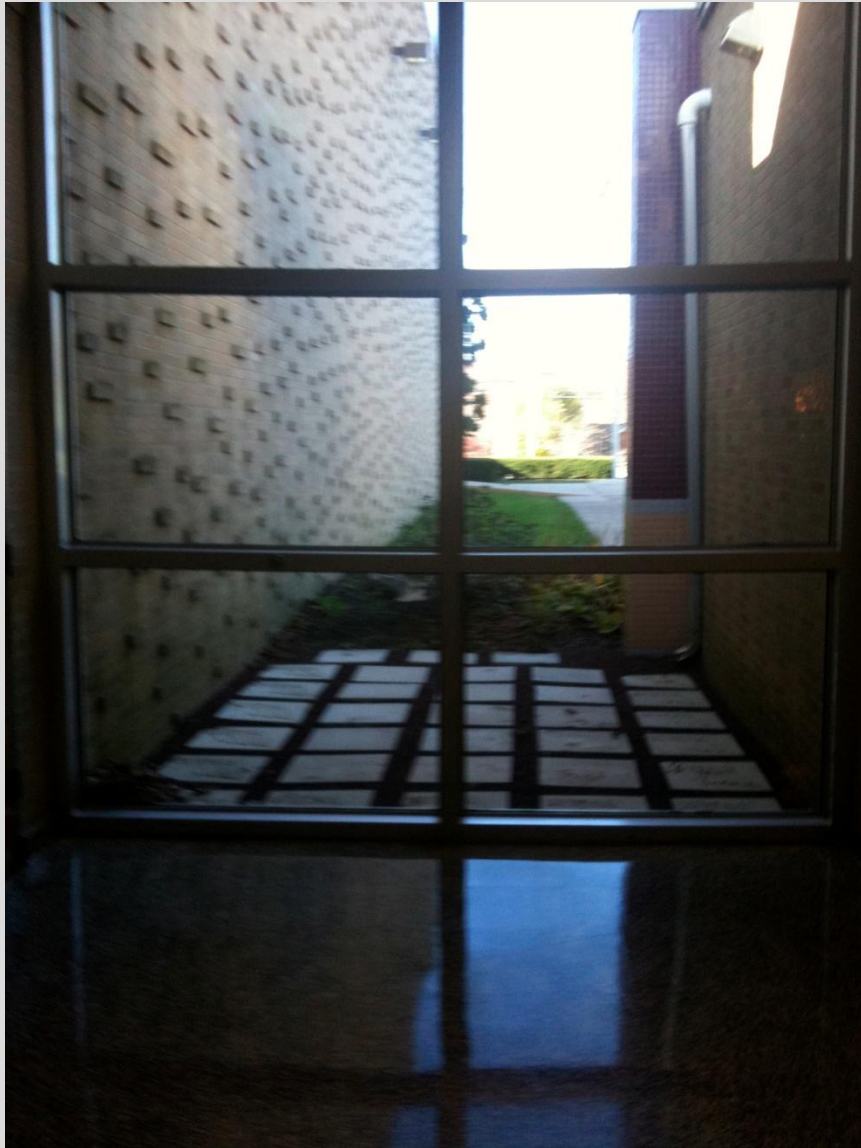
Single Pane Glass/Aluminum Frame at Main Entrance
