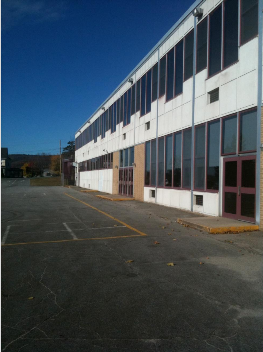
Typical Exterior Dryvit Panels Installed Over Metal Sheeting
