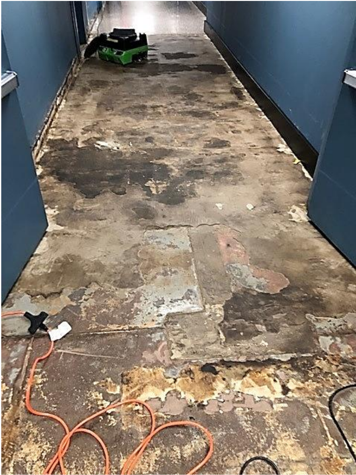
PHOTO 3: POST ASBESTOS ABATEMENT FLOOR PATCH IN CORRIDOR BETWEEN CAFETERIA & BOILER ROOM
