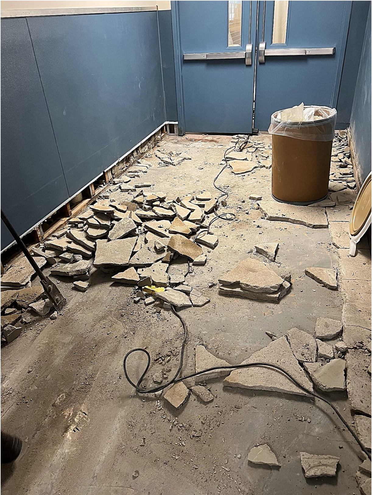
PHOTO 11: REMOVAL OF OVER SLAB BY ENVIRONMENTAL CONTRACTOR – CORRIDOR BETWEEN CAFETERIA & BOILER ROOM
