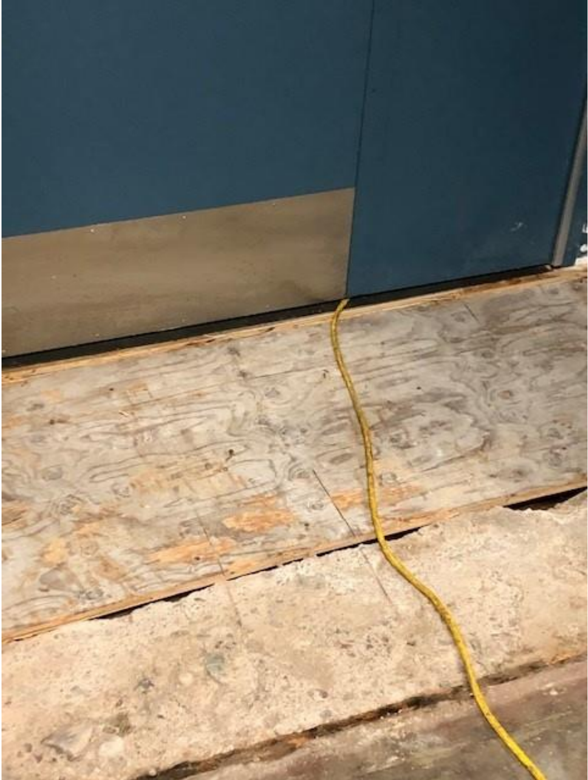
PHOTO 2: WOOD PLANKING AFTER VCT REMOVAL
