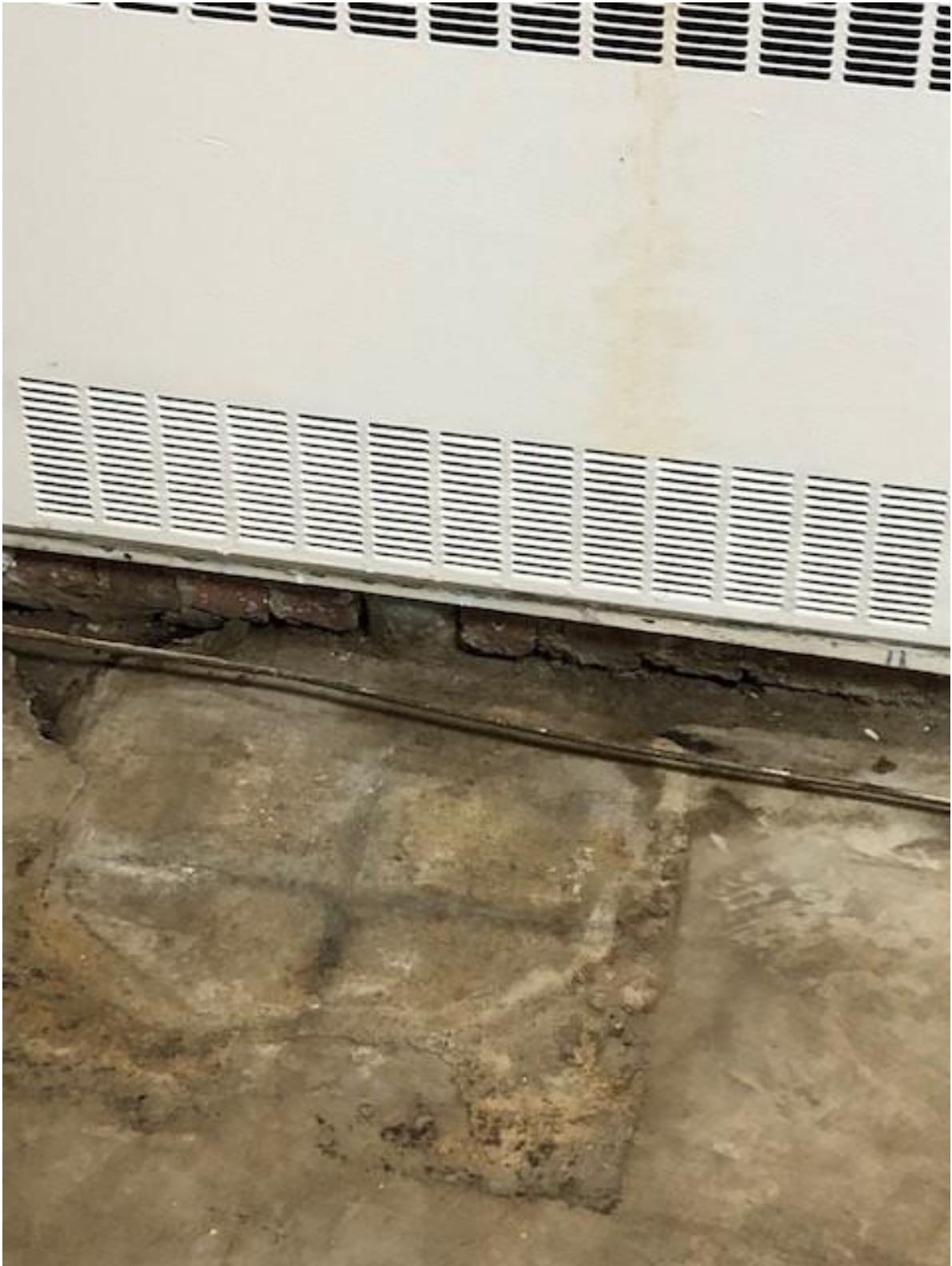
PHOTO 4: POST ASBESTOS ABATEMENT FLOOR & BRICK IN FACULTY ROOM
