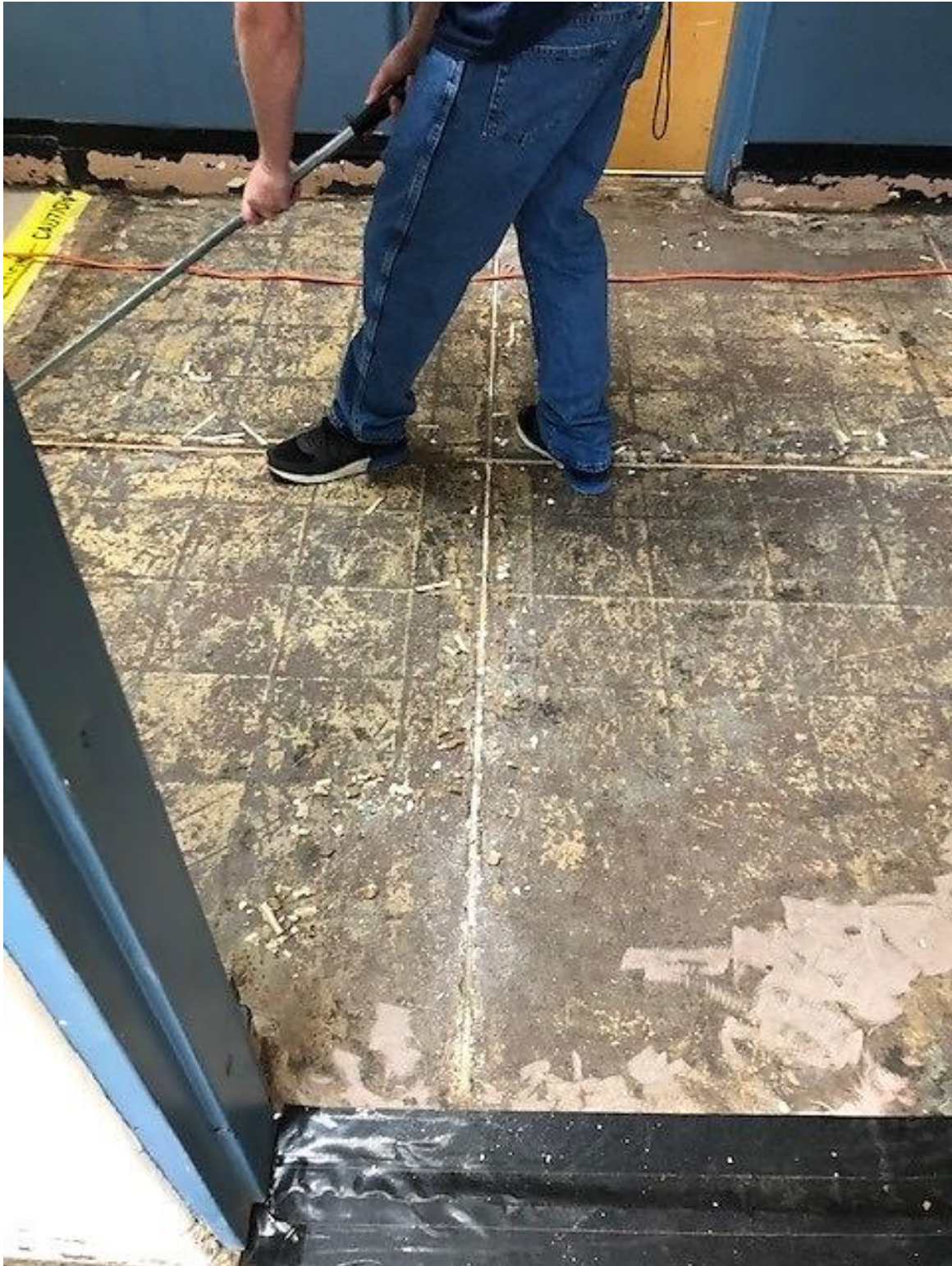
PHOTO 10: DISTRICT STAFF REMOVING FLOOR LEVELER
