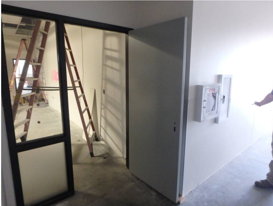
AED and fire extinguisher Cabinets
