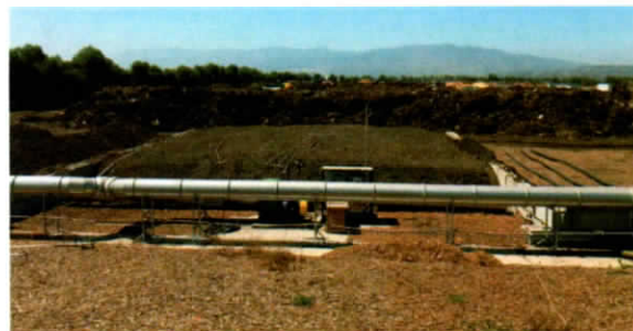
Organics Solutions. CASP System at Agromin OC Chino
