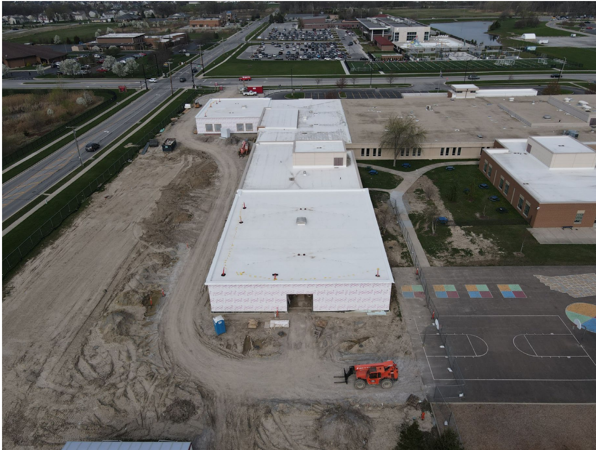
Unit D Classroom Addition
