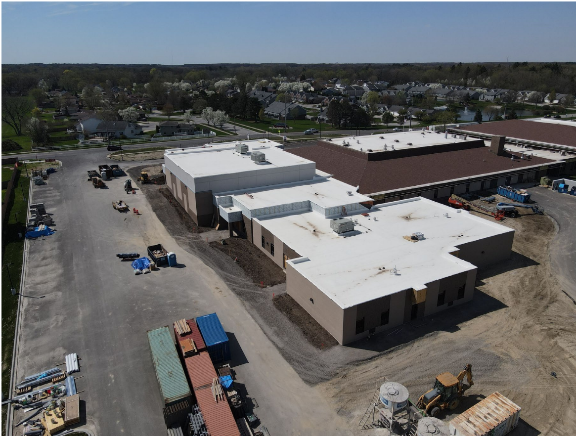
East Side Sidewalk Prep
