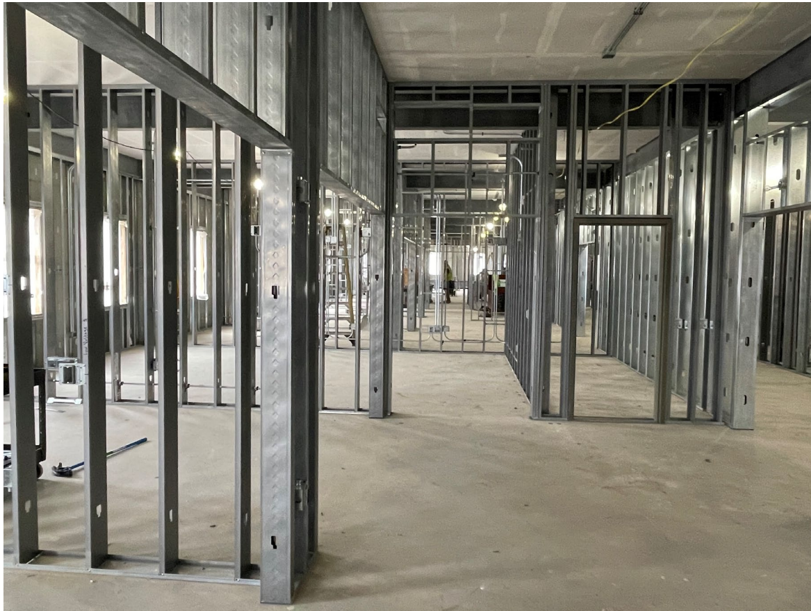
Second Floor Interior Metal Stud Framing
