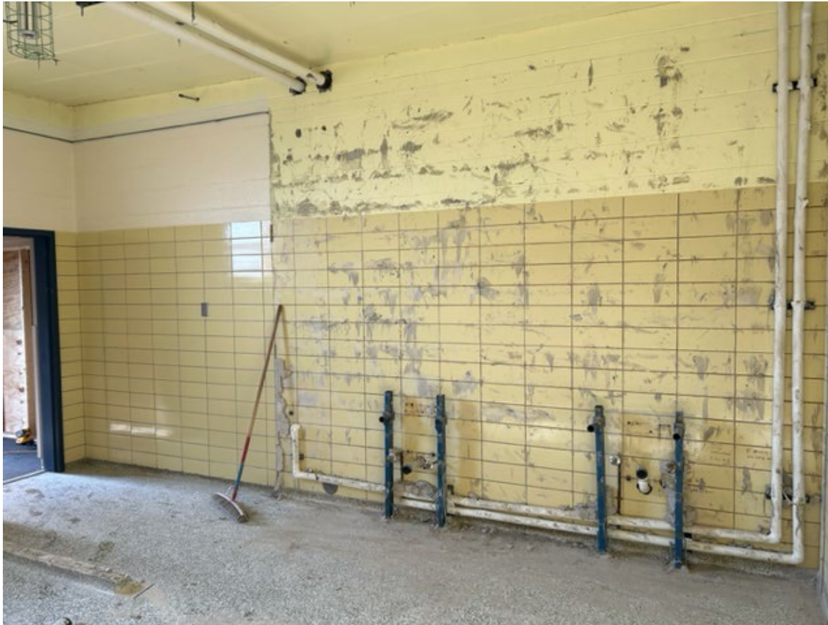
Unit B Restroom Demolition
