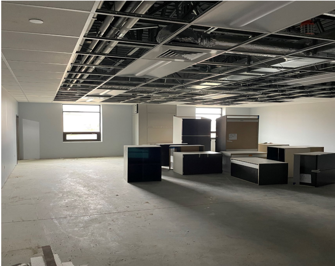
Classroom Addition Classroom Casework
