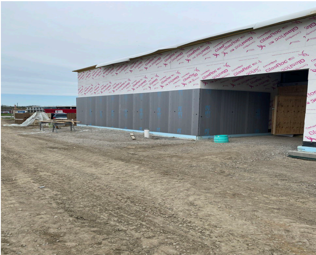
Unit E Classroom Addition Brick Prep
