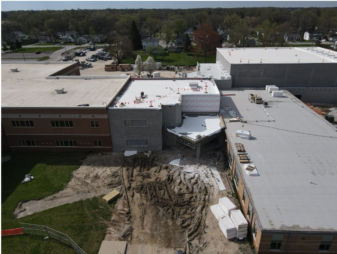
Classroom Addition Exterior CMU
