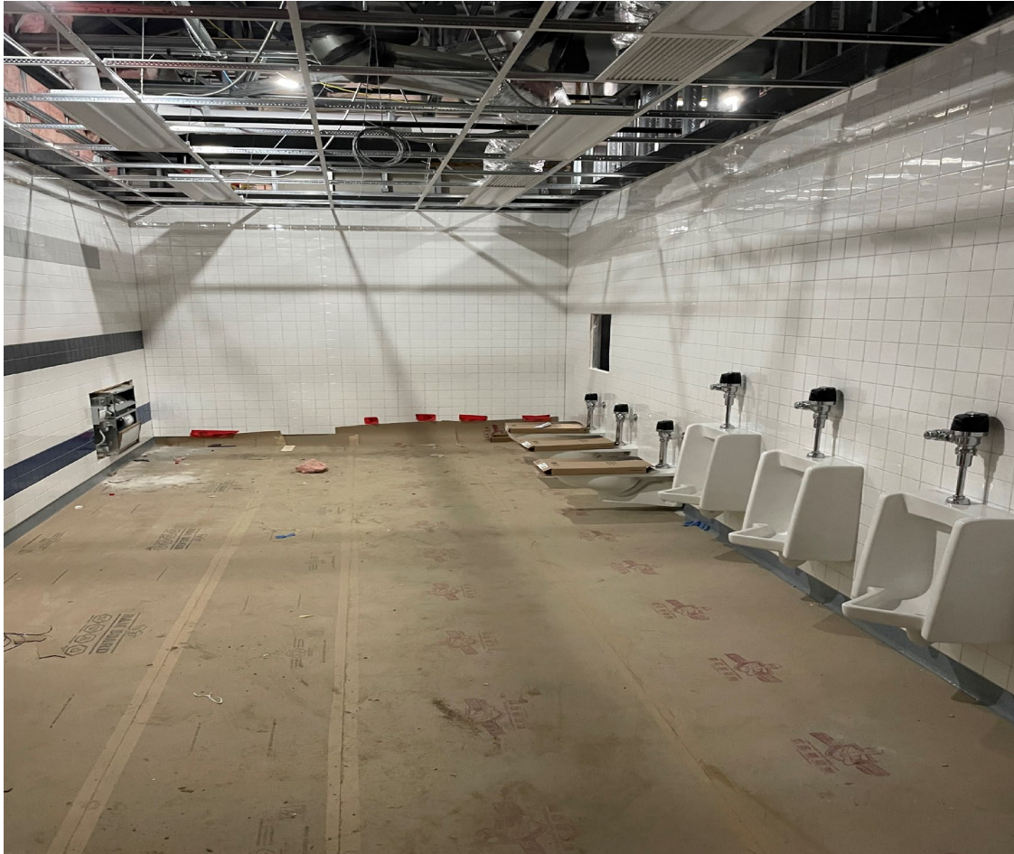
Classroom Addition Restrooms
