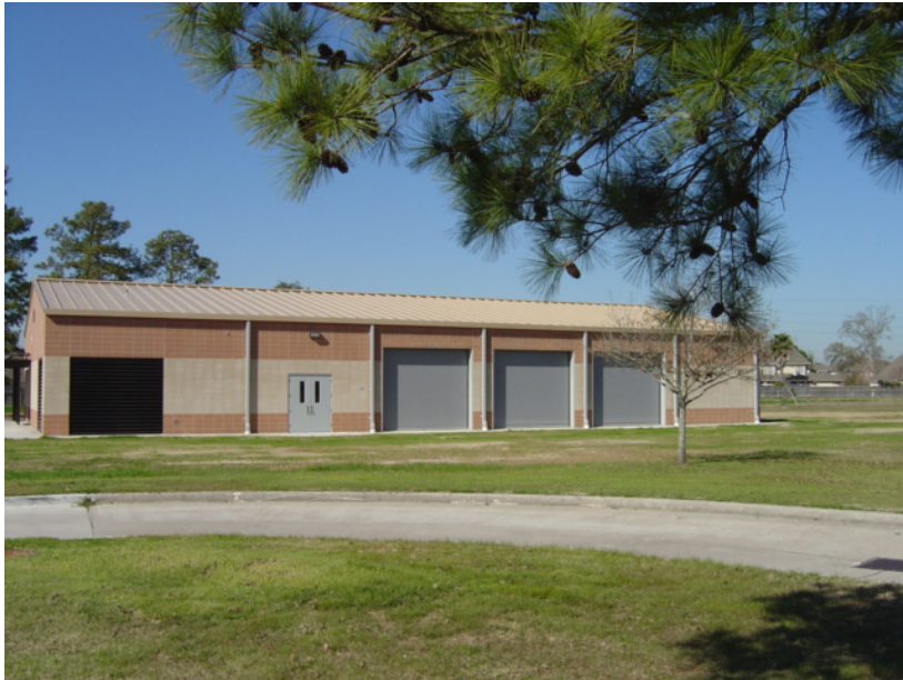
PE Facility constructed with 2004 Bond Funds.
