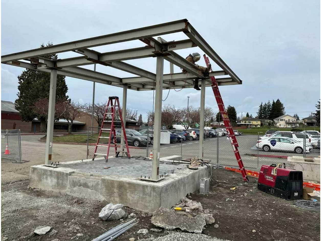
Structural steel assembly at the new athletics field's ticket booth
