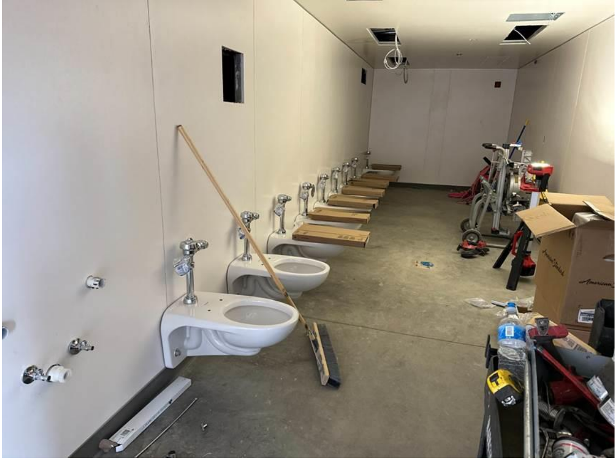
Toilets installed in the Grandstands' restrooms
