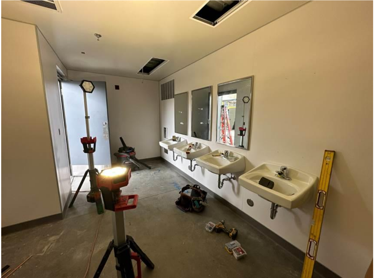
Sinks installed in the Grandstands' restrooms
