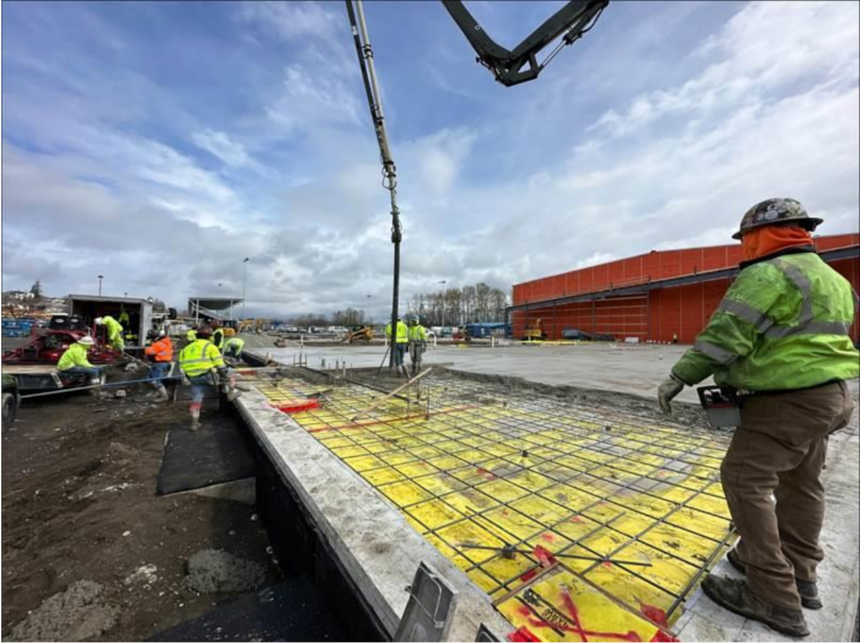
New CTE Wing floor slab being poured
