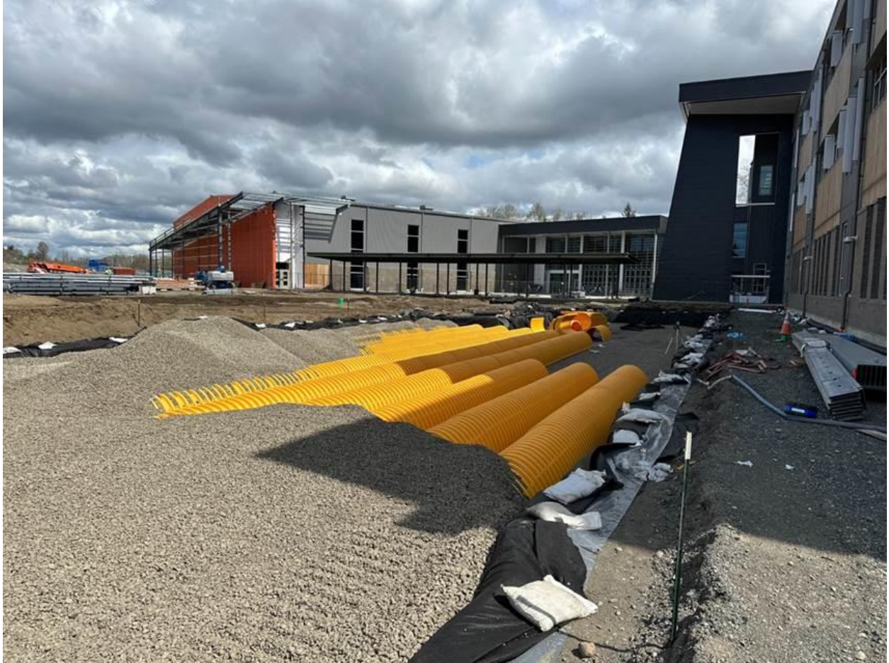
Underground stormwater detention system's ongoing installation
