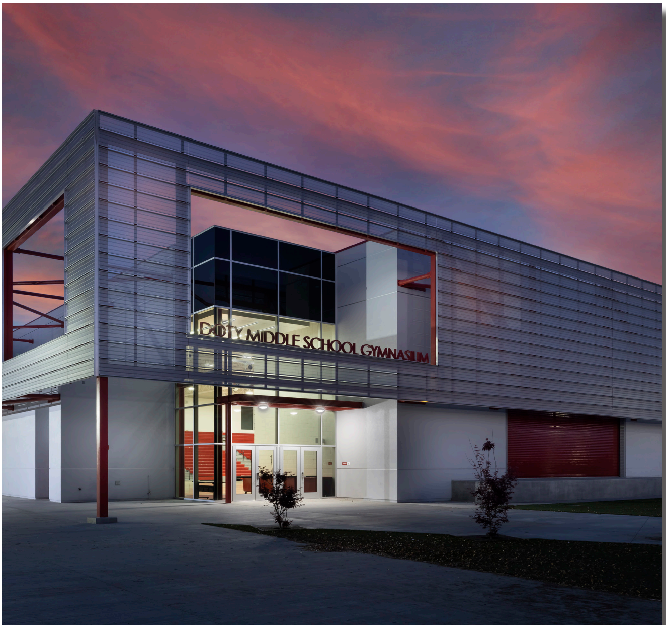
DOTY MIDDLE SCHOOL MODERNIZATION
