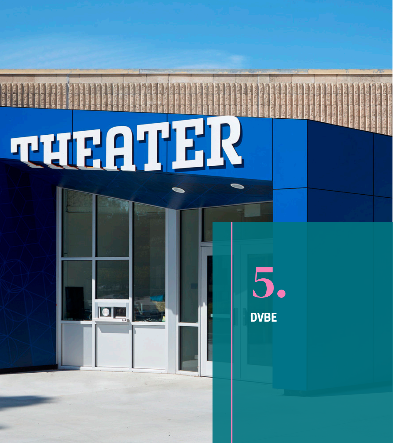
San Diego Unified School District Mira Mesa High School Music Building
