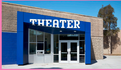
SAN DIEGO UNIFIED SCHOOL DISTRICT Mira Mesa High School Music Buildings
