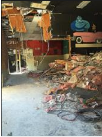
Partial demolition of the Lincoln High School 1200 wing building
