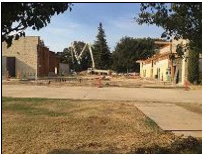
New footings being poured at the Lincoln High School 1200 wing building
