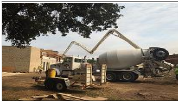
New footings being poured at Lincoln High School
