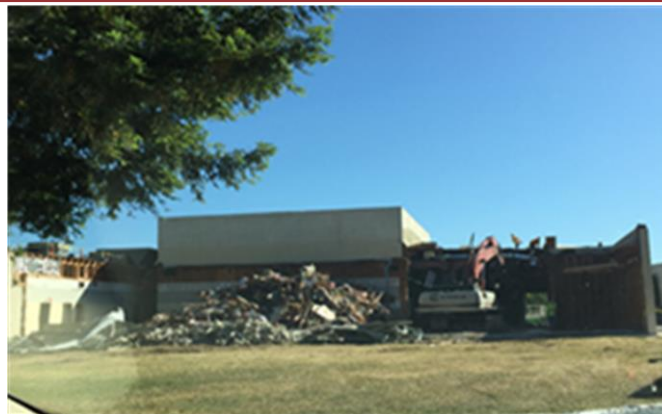
The partial demolition of the Lincoln High School 1200 wing building
