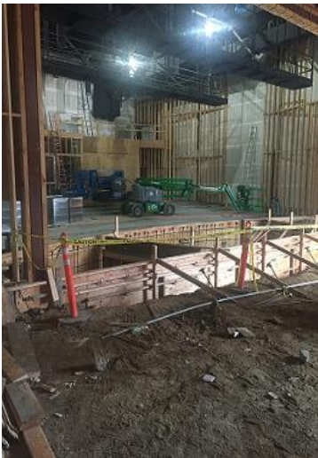
Building the orchestra pit inside the Performing Arts Center
