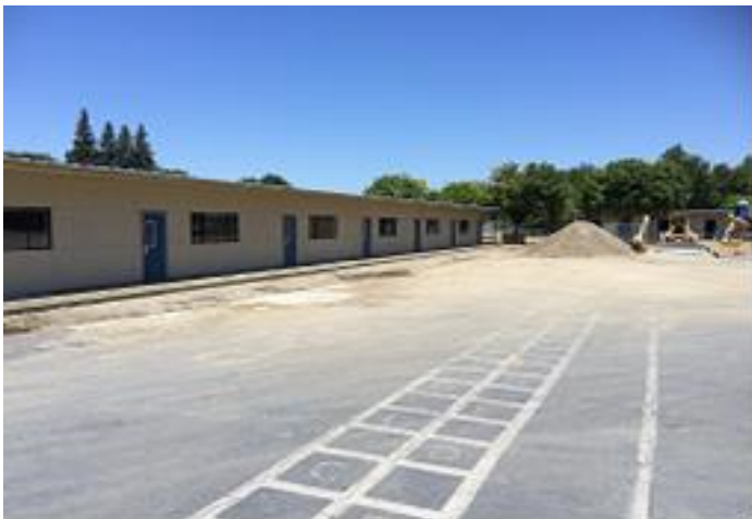
Claudia Landeen School new modular wing completed August 2016
