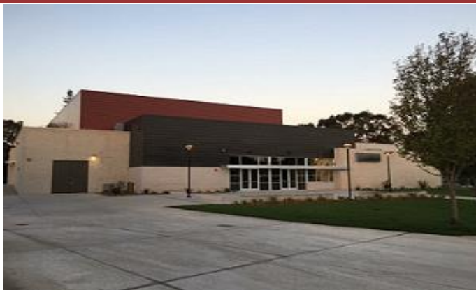
The "before" and "after" of the Lincoln High School Performing Arts Center
