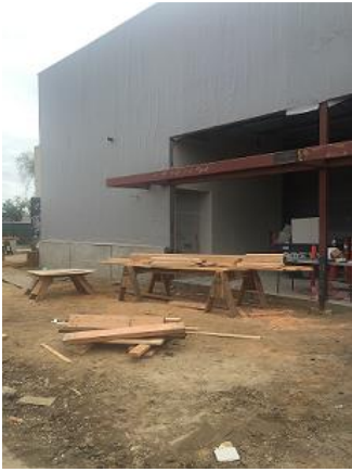
Renovation of the Lincoln High School Performing Arts Center
