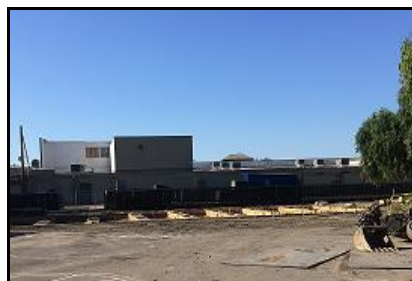
New foundations for the new classrooms at Lincoln Elementary School
