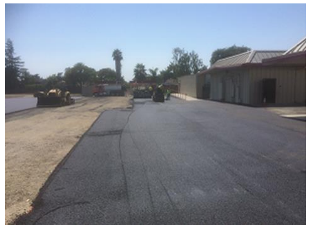
New asphalt at Mable Barron School
