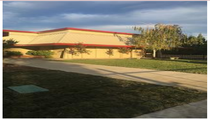
Claudia Landeen School and Mable Barron School modernization projects
