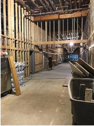
Renovation of the Mable Barron School main building
