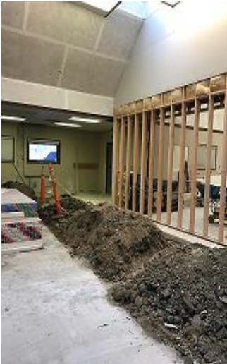
Renovation of a classroom in the Claudia Landeen School main building
