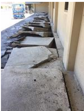
Replacement of sidewalks at Claudia Landeen School
