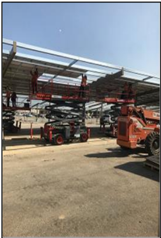
Installation of new solar panels at Lincoln High School
