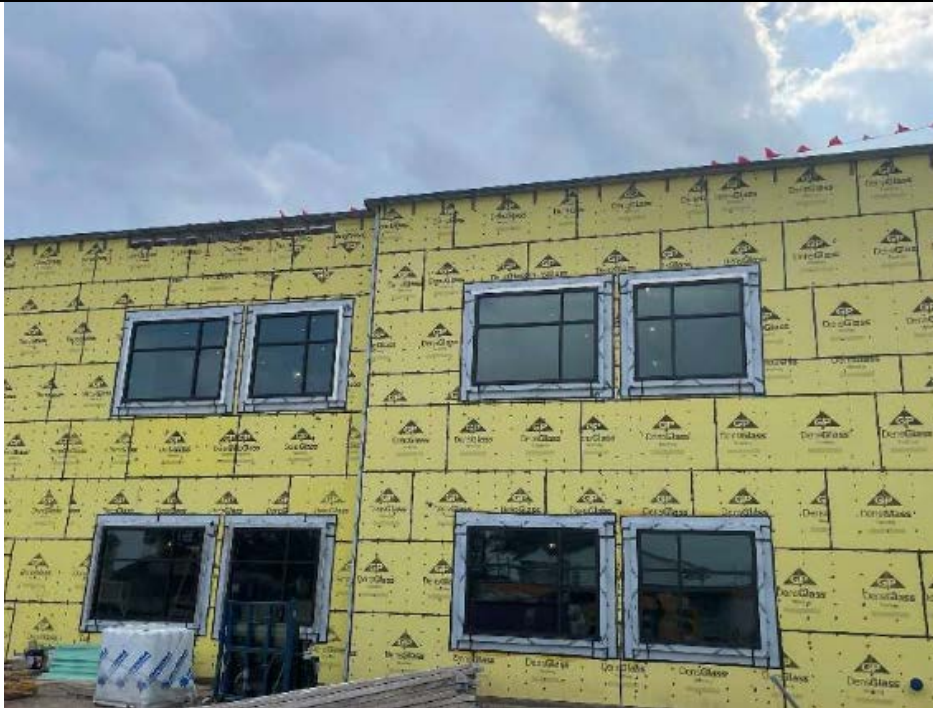
Glazing installation
