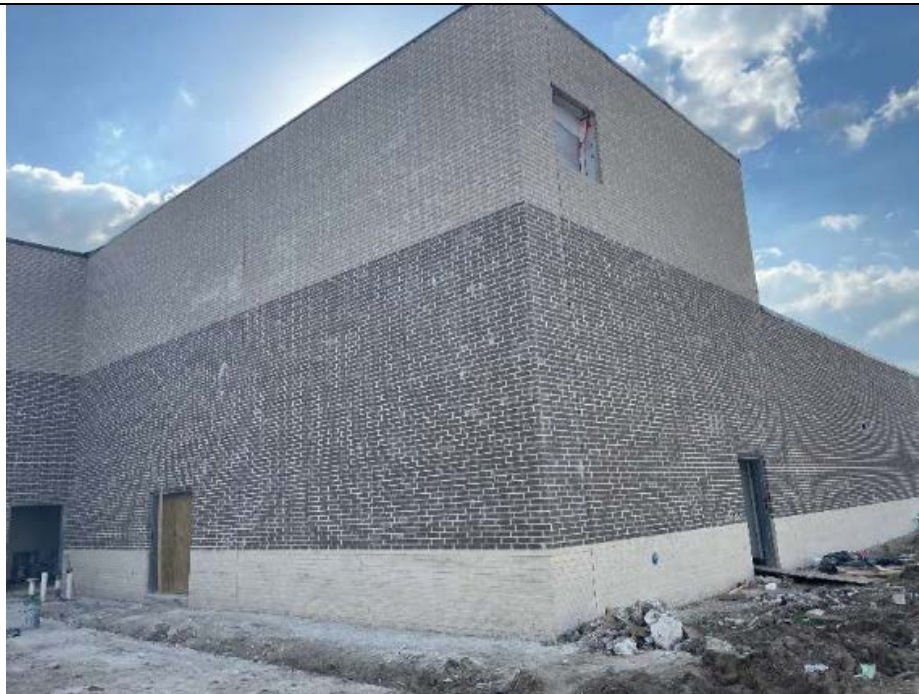
Area D brick installation
