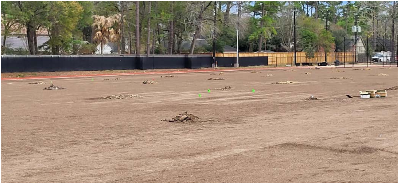
Playfield Irrigation installation
