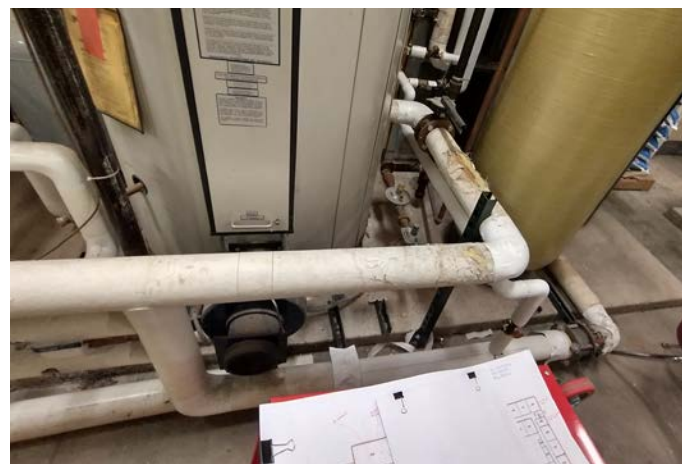
DAMAGED INSULATION
