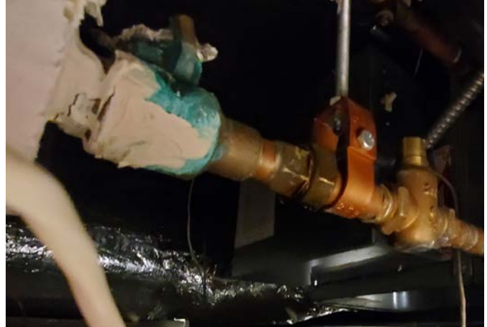
VALVE ACTUATOR REMOVED FROM VALVE BODY
