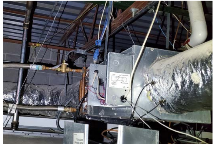
REMOVED HEATING VALVE ACTUATOR ON VAV
