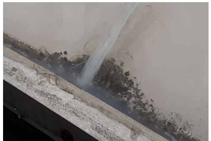
CAULKING AT CRACKED SKYLIGHT
