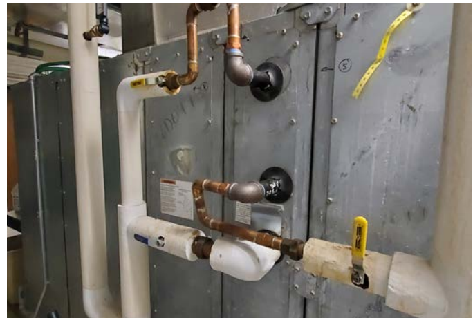
AHU-4 HOT WATER COIL REPAIR IN PROGRESS
