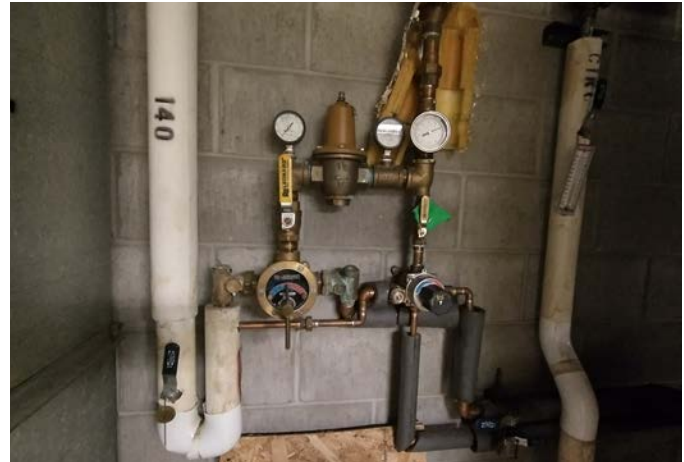
THERMOSTATIC MIXING VALVE
