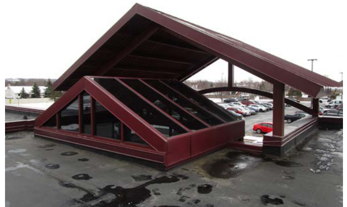
SKYLIGHT ABOVE ENTRY VESTIBULE
