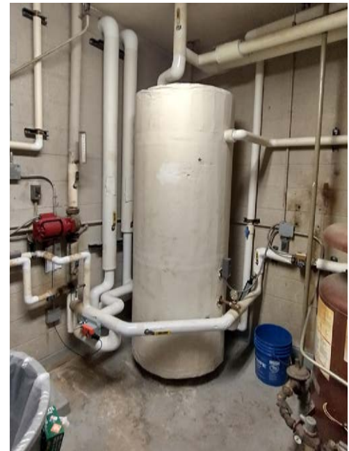
NORTH STORAGE TANK
