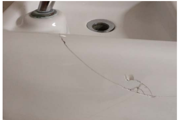
CRACKED DRINKING FOUNTAIN
