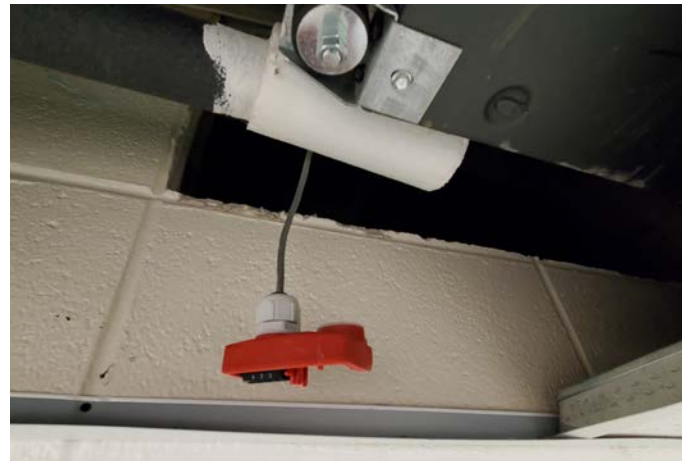
HEAT PUMP VALVE ACTUATOR WIRING HARNESS REMOVED
