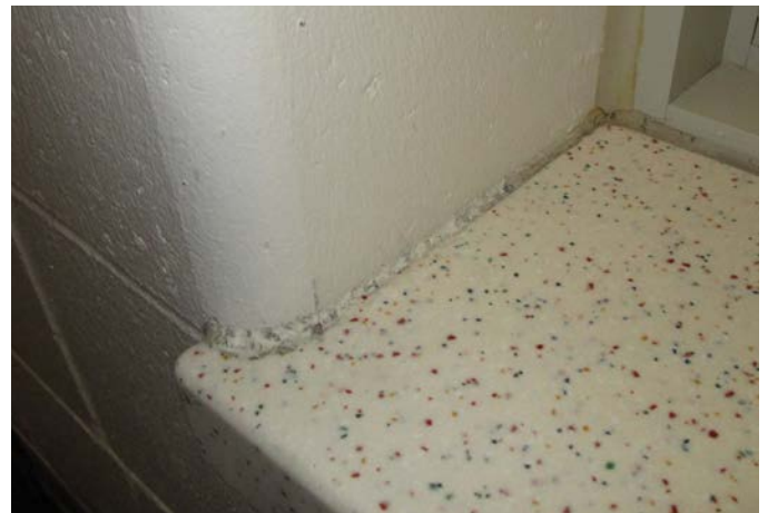
INTERIOR WINDOW SILL SEALANT JOINT
