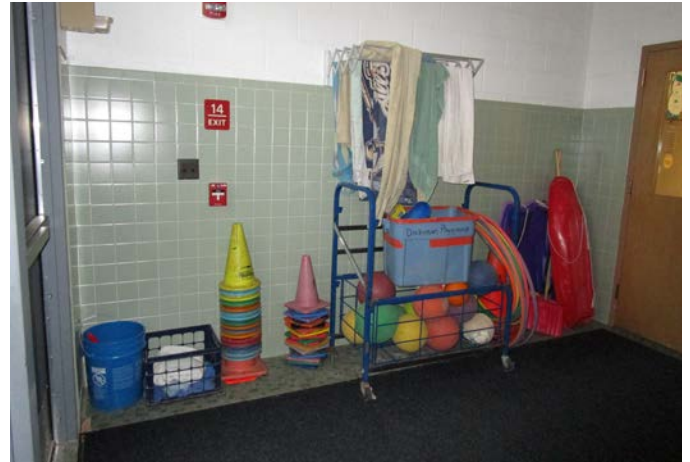
EXIT VESTIBULE USED TO STORE PLAYGROUND EQUIPMENT
