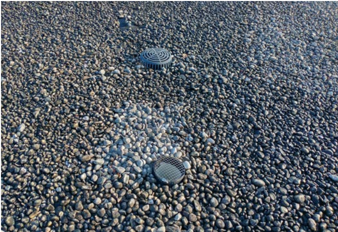
ROOF DRAIN WITH OVERFLOW
