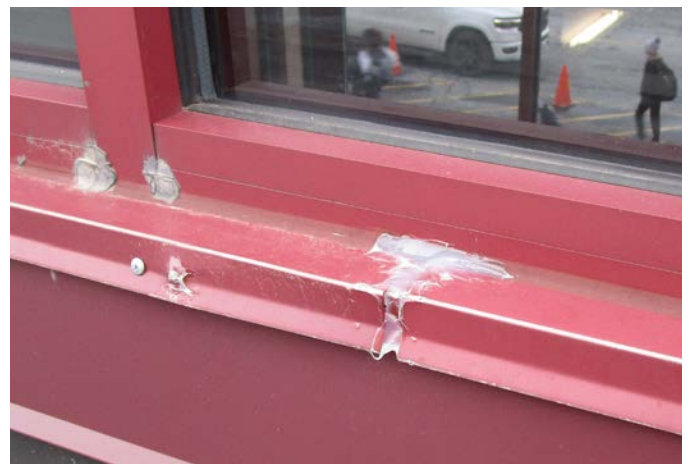
SEALANT APPLIED TO EXTERIOR OF WINDOW SILL
