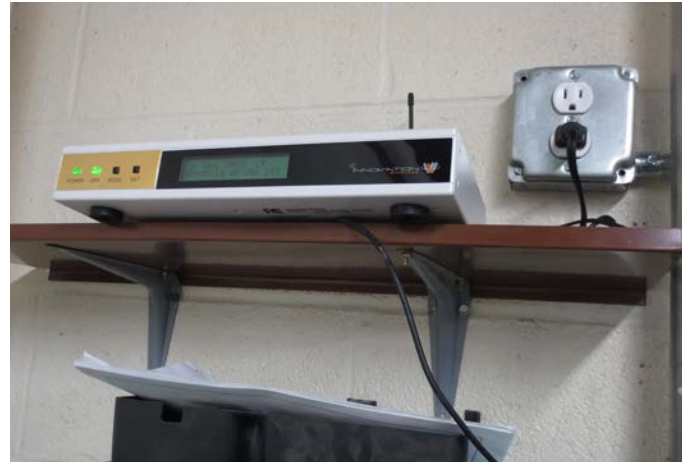
WIRELESS CLOCK TRANSMITTER
