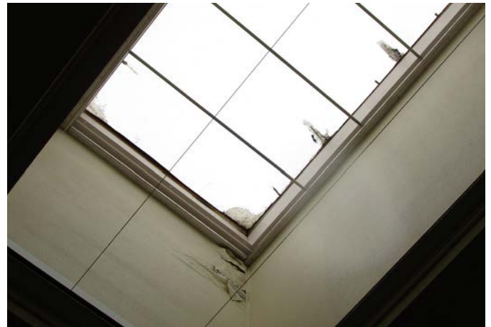
INTERIOR OF SKYLIGHT WELL
