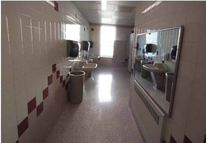
TYPICAL STUDENT RESTROOMS
