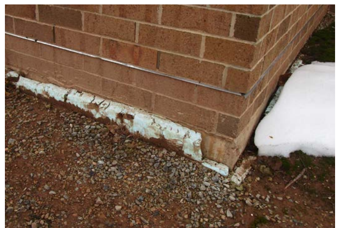
EXPOSED EXTERIOR WALL INSULATION
