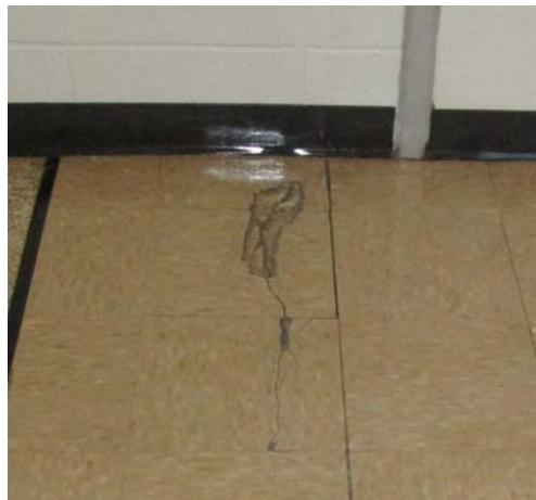
VCT FLOORING THAT CROSSES A BUILDING JOINT, THAT HAS NOW CRACKED
