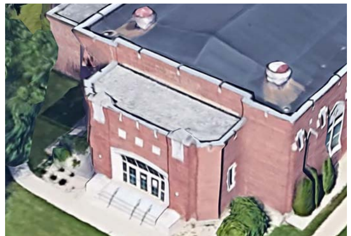
VIEW OF AUDITORIUM BALCONY ROOF
