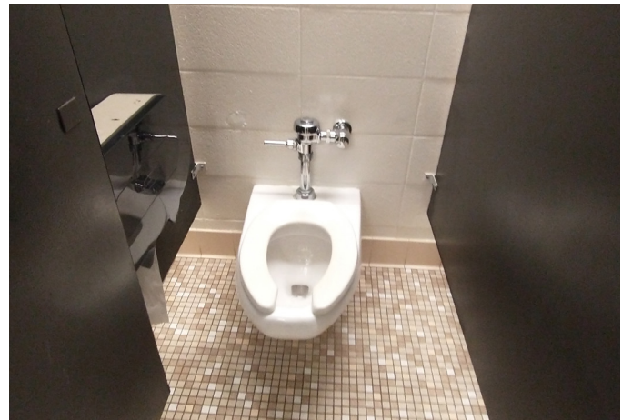
ORIGINAL WATER CLOSET
