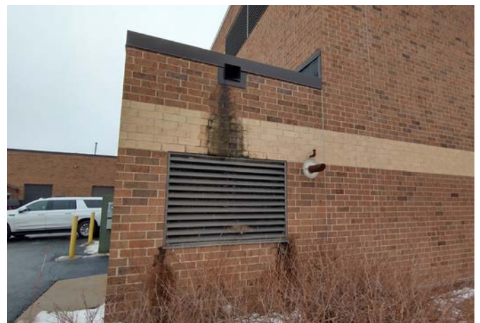
GENERATOR ENCLOSURE ROOF SCUPPER
