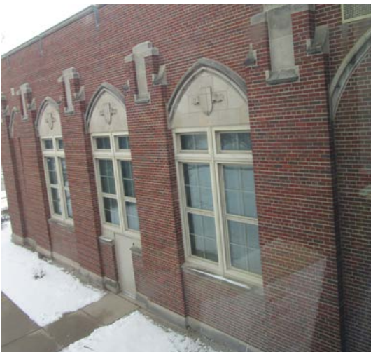
EXTERIOR VIEW OF THE AUDITORIUM, AND A CONSTRUCTION DOCUMENT FROM SPECIALTY ENGINEERING GROUP NOTING WORK TO REPLACE SEALANT, TUCKPOINTING MORTAR JOINTS, REPLACING LIMESTONE TRIM, AND RE-GASKETING WINDOW SEALS.
