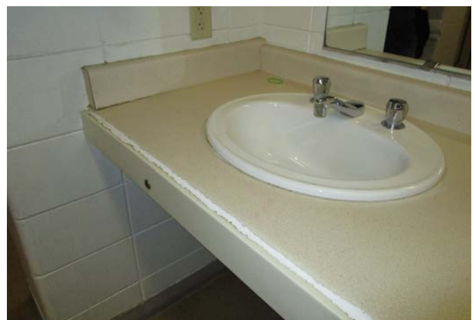
LOCKER ROOM VANITY
