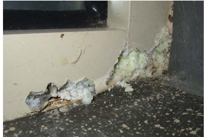
AT THE NORTHEAST ENTRY ALUMINUM DOORS
