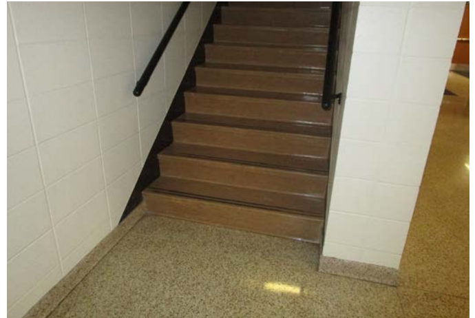
STAIRS COVERED WITH VINYL
