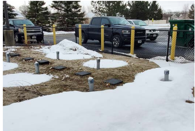
ABANDONED THERMAL STORAGE TANKS
