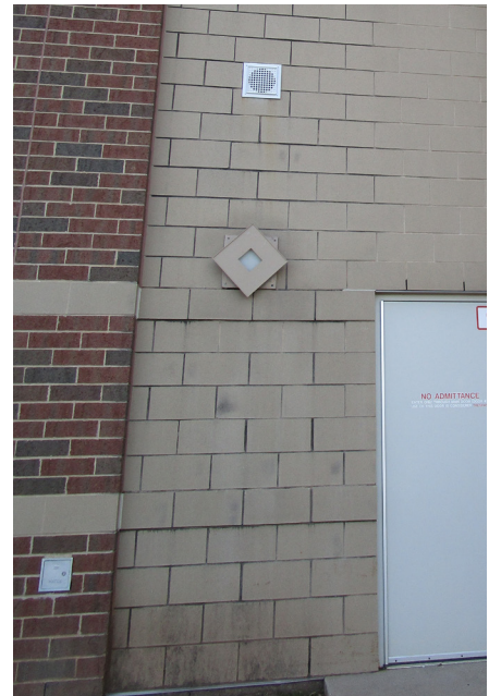
TWO LOCATIONS OF STAINING FROM ROOF OVERFLOW WATER
