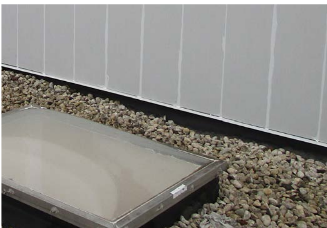
CAULKING USED TO SEAL METAL WALL PANELS
