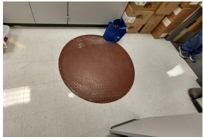
ACID NEUTRALIZATION BASIN
