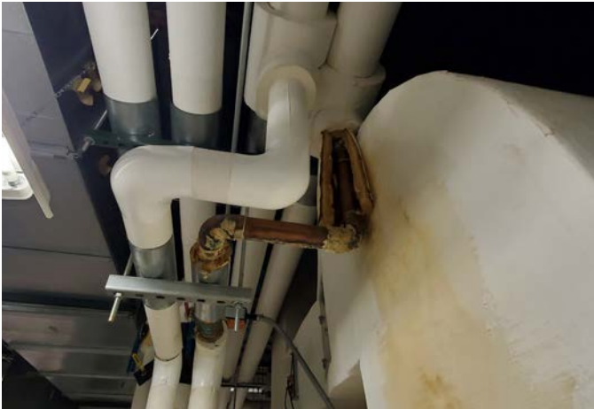
TYPICAL LEAK REPAIR ON HOT WATER PIPING
