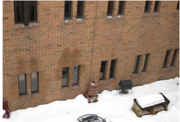
ORIGINAL WINDOWS YET TO BE REPLACED IN THE COURTYARD
