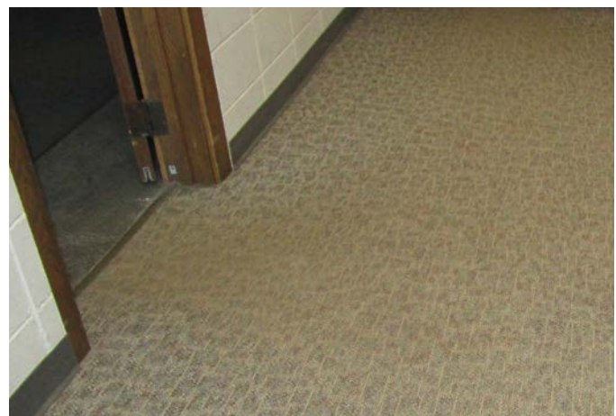
CARPET AT MAIN OFFICE ENTRANCE
