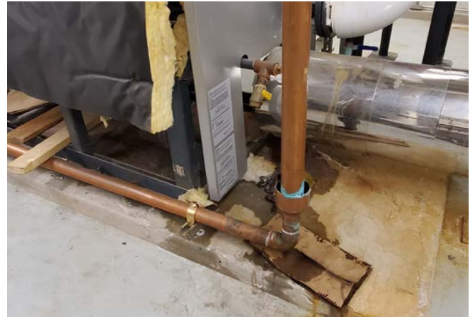
BOILER UNDER REPAIR FOR CRACKED HEAT EXCHANGER
