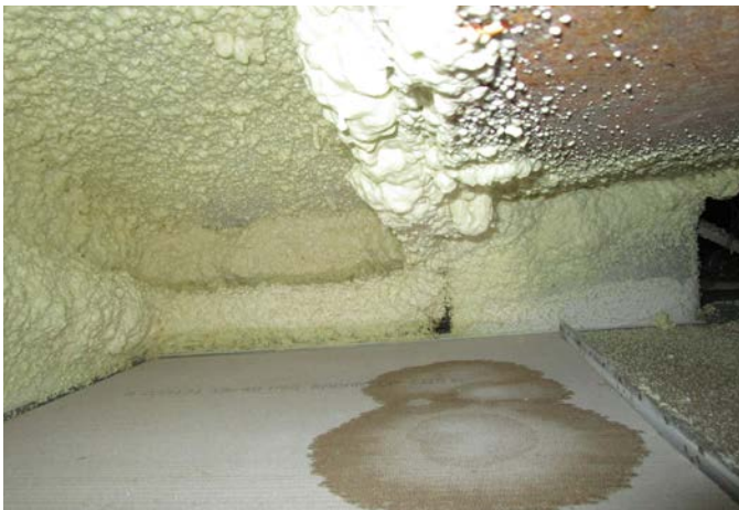
SPRAY FOAM INSULATION
