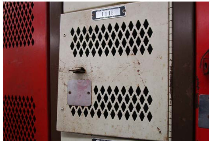
RUST ON ORIGINAL 1976 LOCKERS
