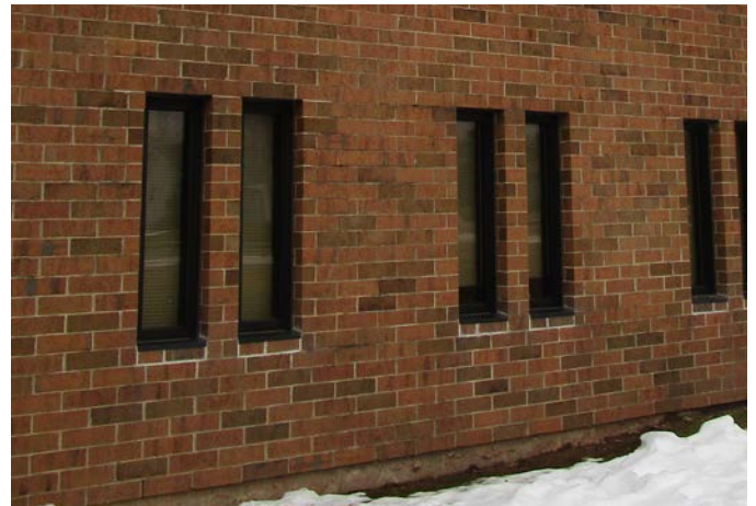
REPLACEMENT WINDOWS WITH NEW SILLS
