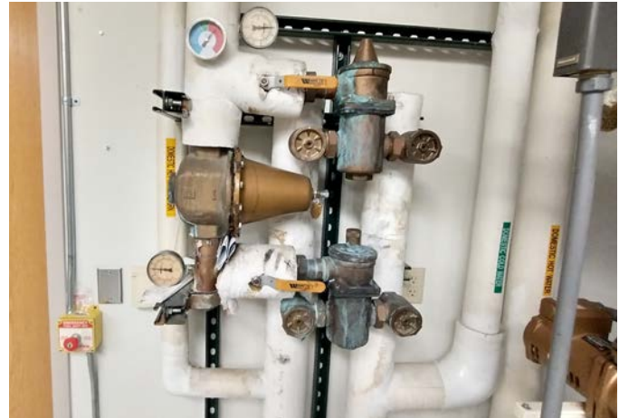
THERMOSTATIC MIXING VALVE
