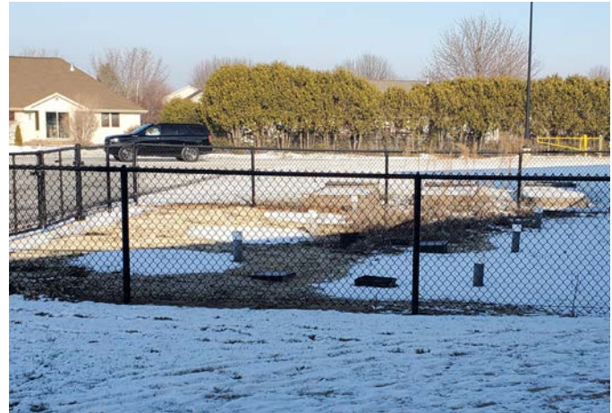
ABANDONED THERMAL STORAGE TANKS
