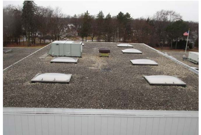
SKYLIGHTS ON ROOF ABOVE CAFETERIA
