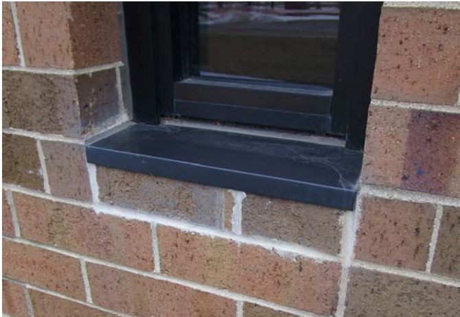
FLAT WINDOW SILLS AT REPLACEMENT WINDOWS
