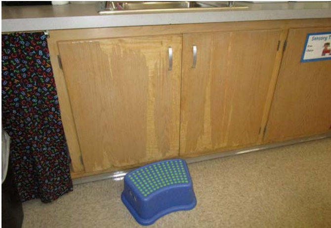
1958 CASEWORK DOORS AT SINKS
