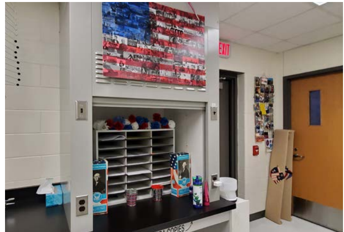
SCIENCE ROOM FUME HOOD NO LONGER USED
