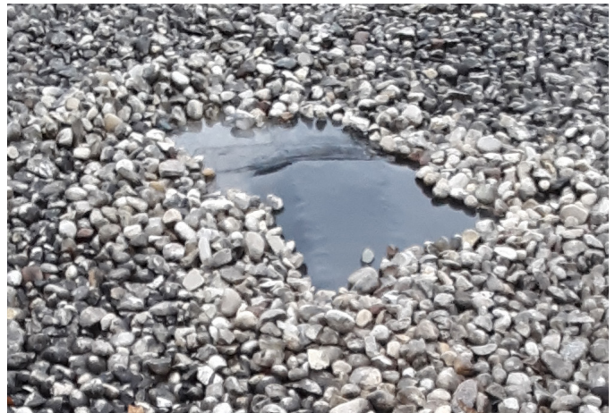
RAISED INSULATION PUSHING UP ON MEMBRANE
