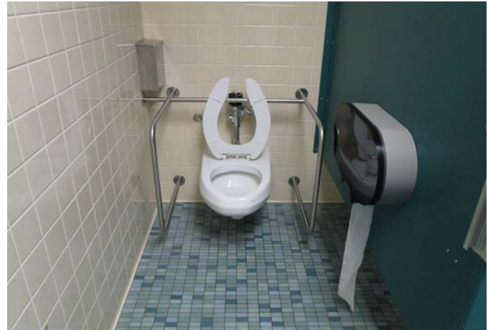
TOILET STALL IN STUDENT RESTROOM
