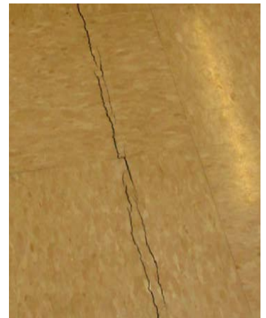
VCT FLOORING THAT CROSSES A BUILDING JOINT, THAT HAS NOW CRACKED
