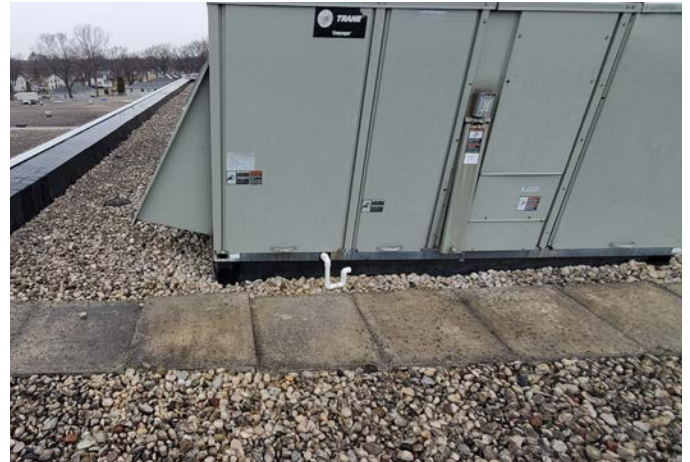
LOW CLEARANCE TO OUTSIDE AIR INTAKE FROM ROOF
