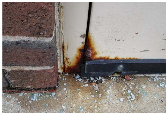
AT THE EAST GYM EXIT DOORS
