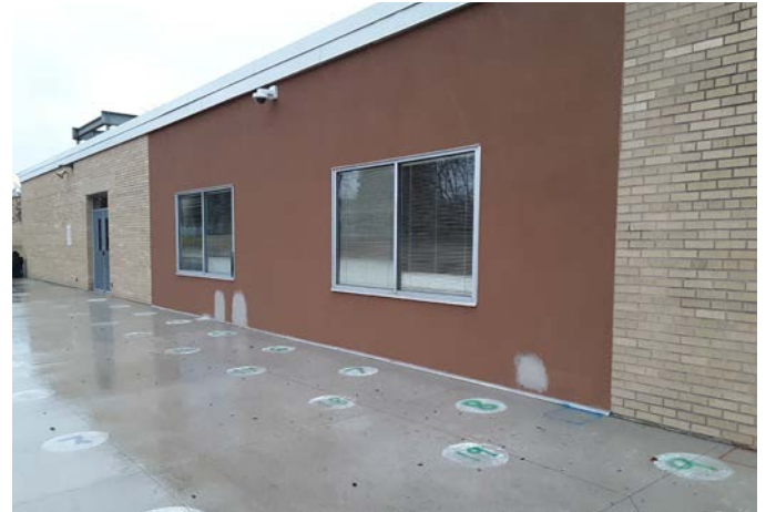
THE 1956 CLASSROOM WINDOW SYSTEM WAS REPLACED WITH NEW WALLS AND SMALLER WINDOWS
