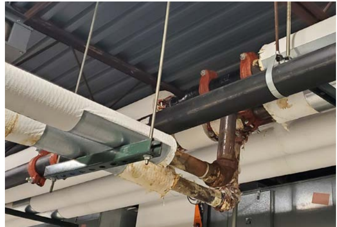
REPAIRED SEGMENT OF LEAKING PIPING
