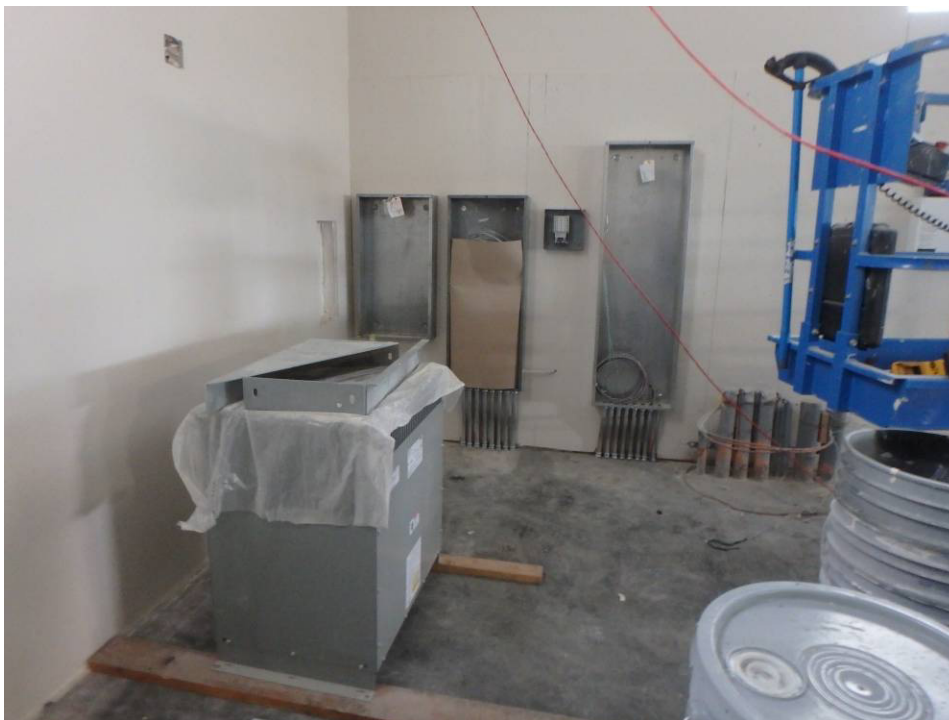
Electrical panels and transformer
