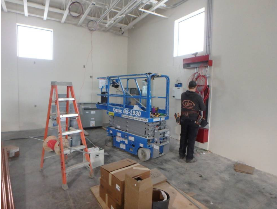
Wiring the fire alarm panel
