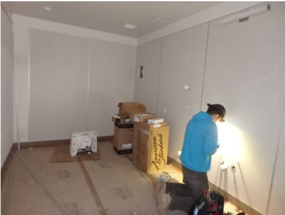
Typical restroom FRP walls
