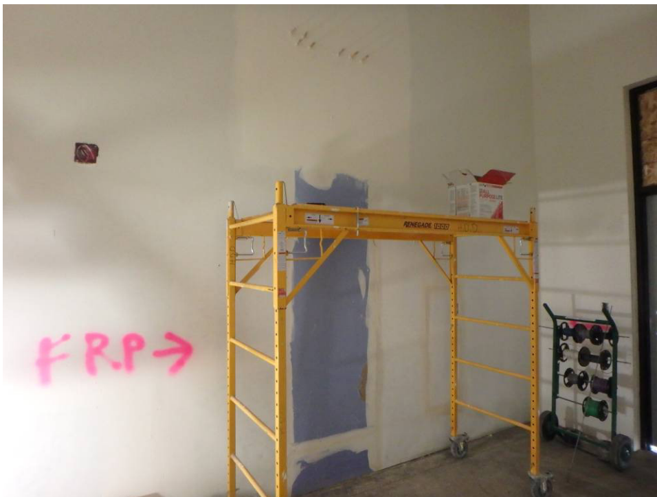
Wallboard repair at the manifold to be relocated in the Kennel Room
