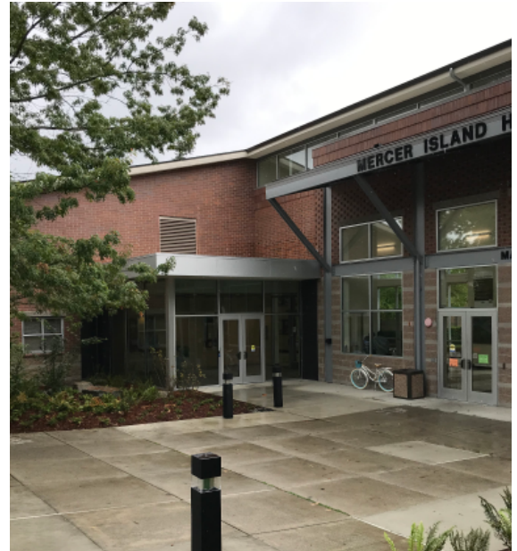
Mercer Island HS: Secure building entry
