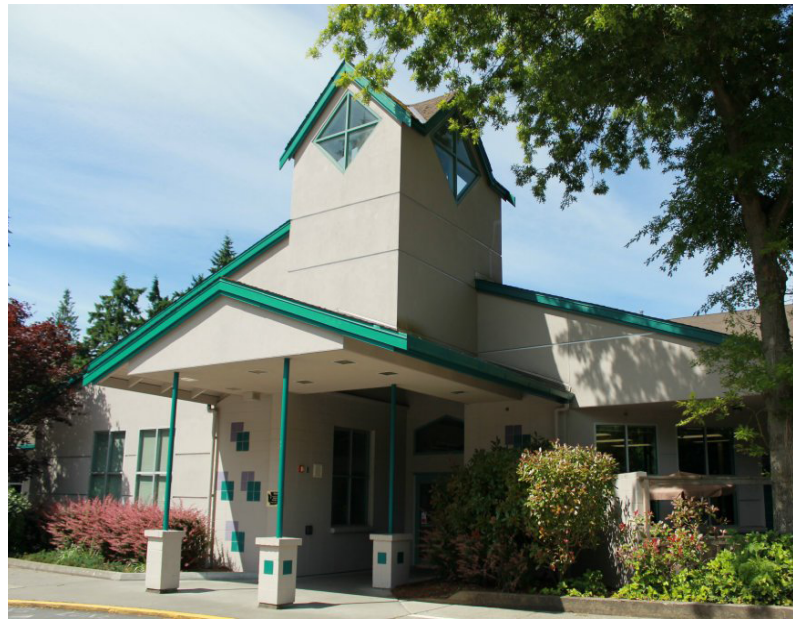
Island Park Elementary School Entry
