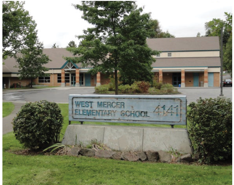
West Mercer Elementary School Entry
