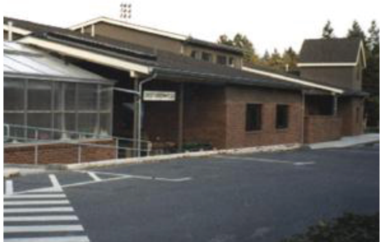
Crest Learning Center Exterior
