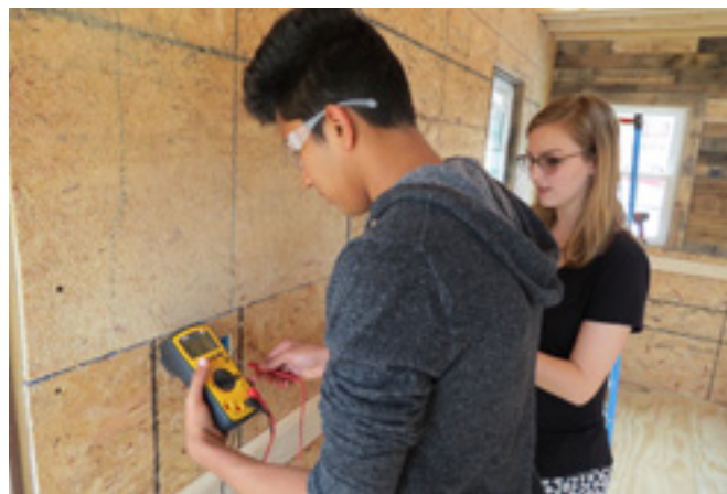
Students run electrical testing on the outlets in the mobile Fab Lab.
