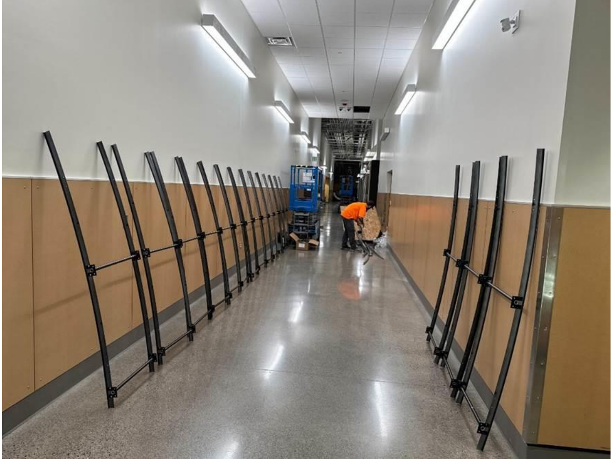
Ceiling cloud installation in the corridors around the gym
