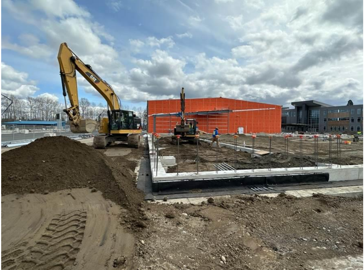
The foundation of the CTE Wing is close to completion
