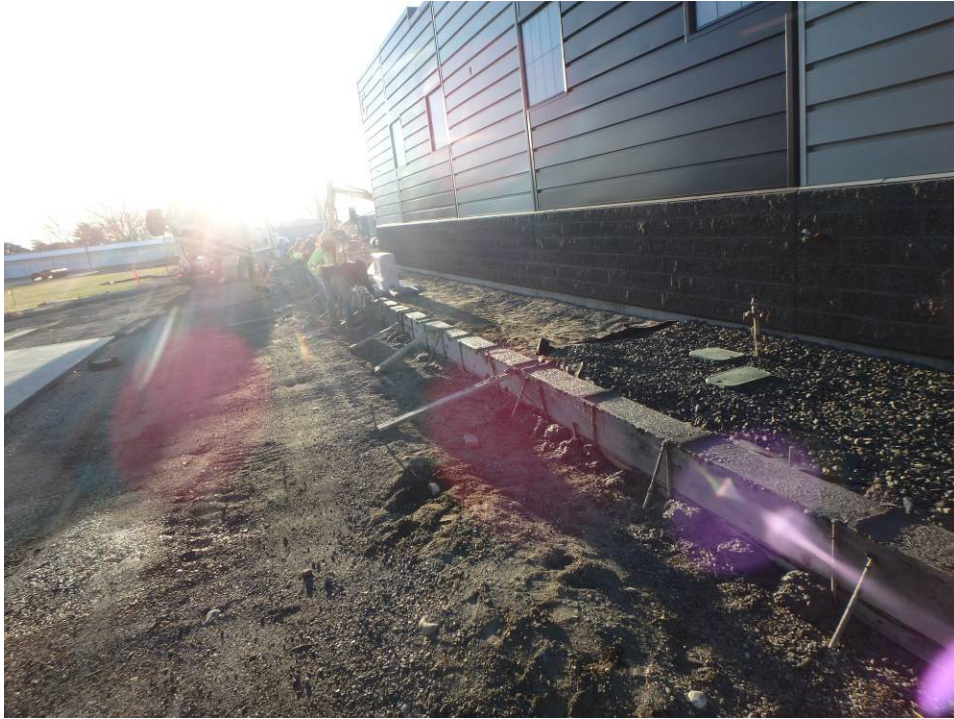
Looking east at the north curb forms and concrete
