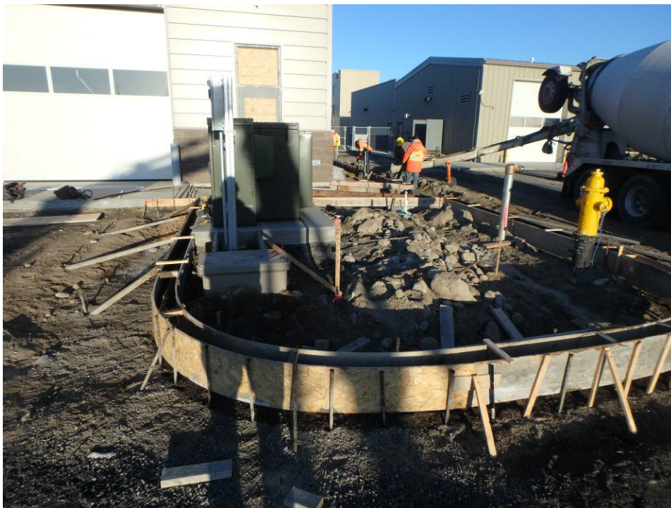
Northeast peninsula formwork
