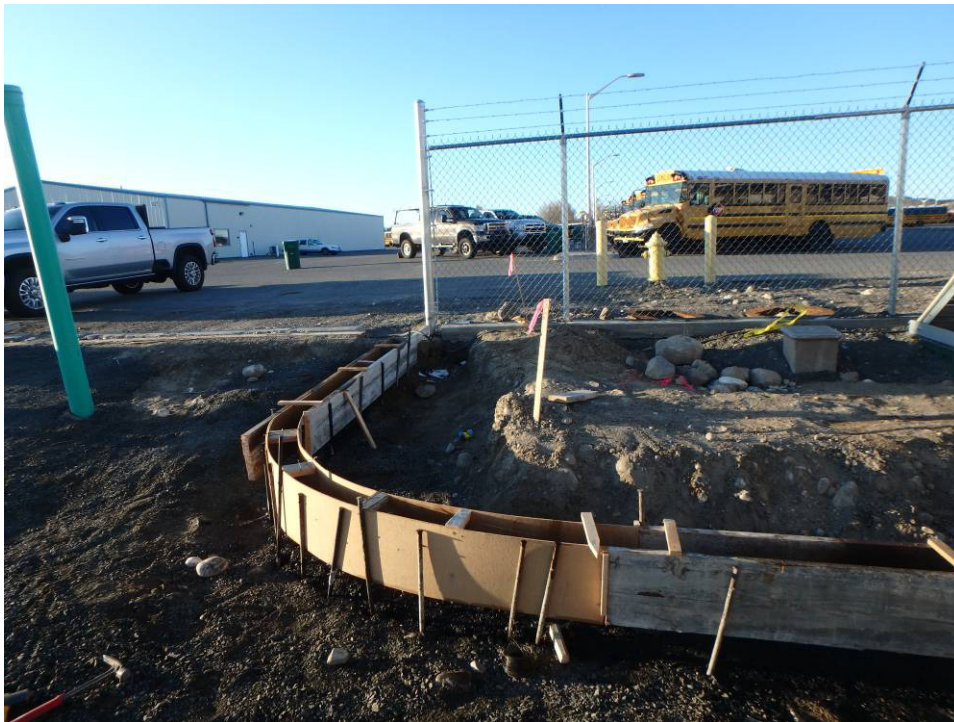
Entry formwork west half
