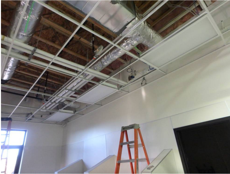
Ceiling grid in the lab – looking southwest
