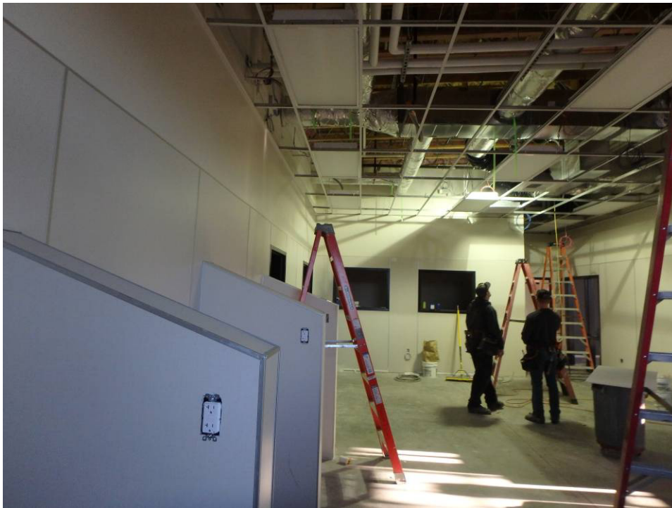
Ceiling grid in the lab – looking north
