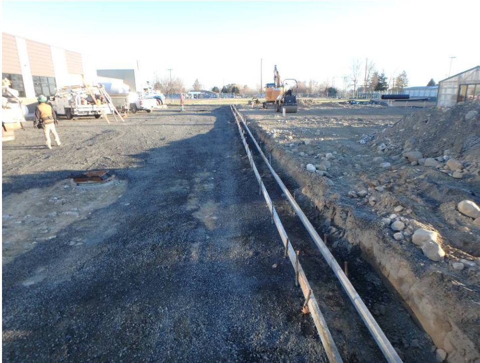
Looking north at the central curb forming
