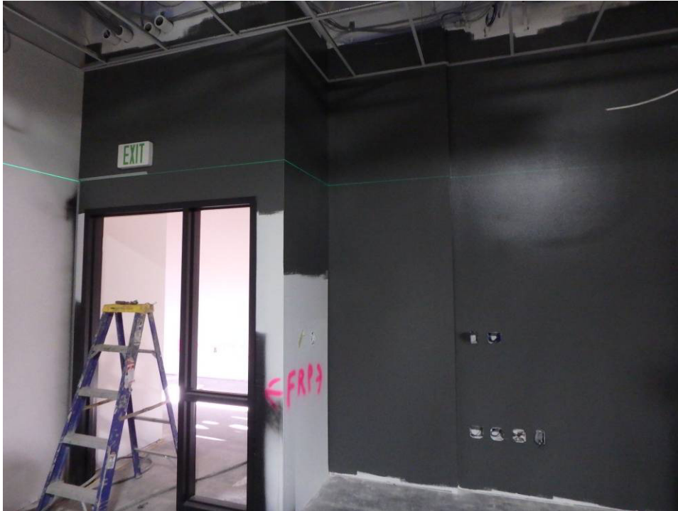
North classroom entry door
