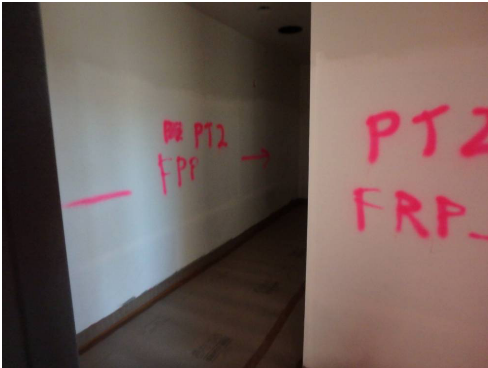
Typical restroom tiling protected
