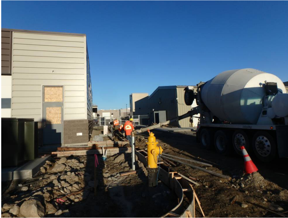
North side of building placing concrete curb
