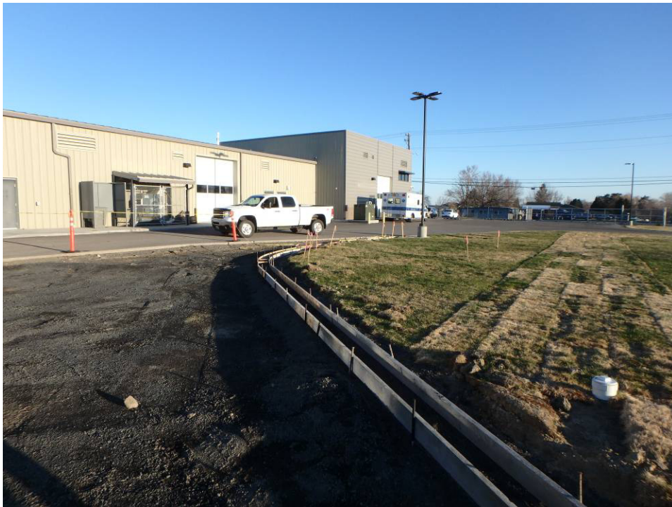
North central site curb forms
