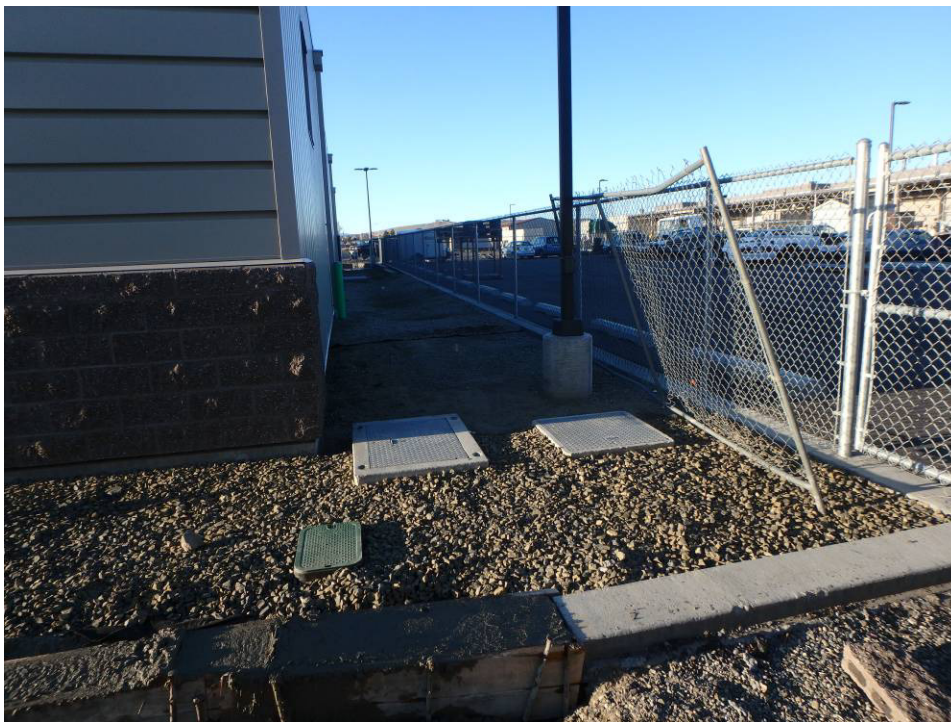
Looking south at the west property line and back of building
