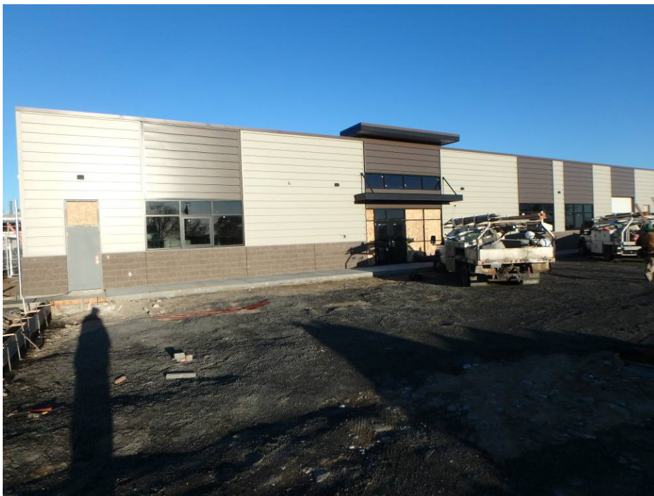
Front entry and sidewalk
