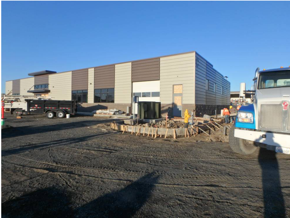
Northeast corner of the building
