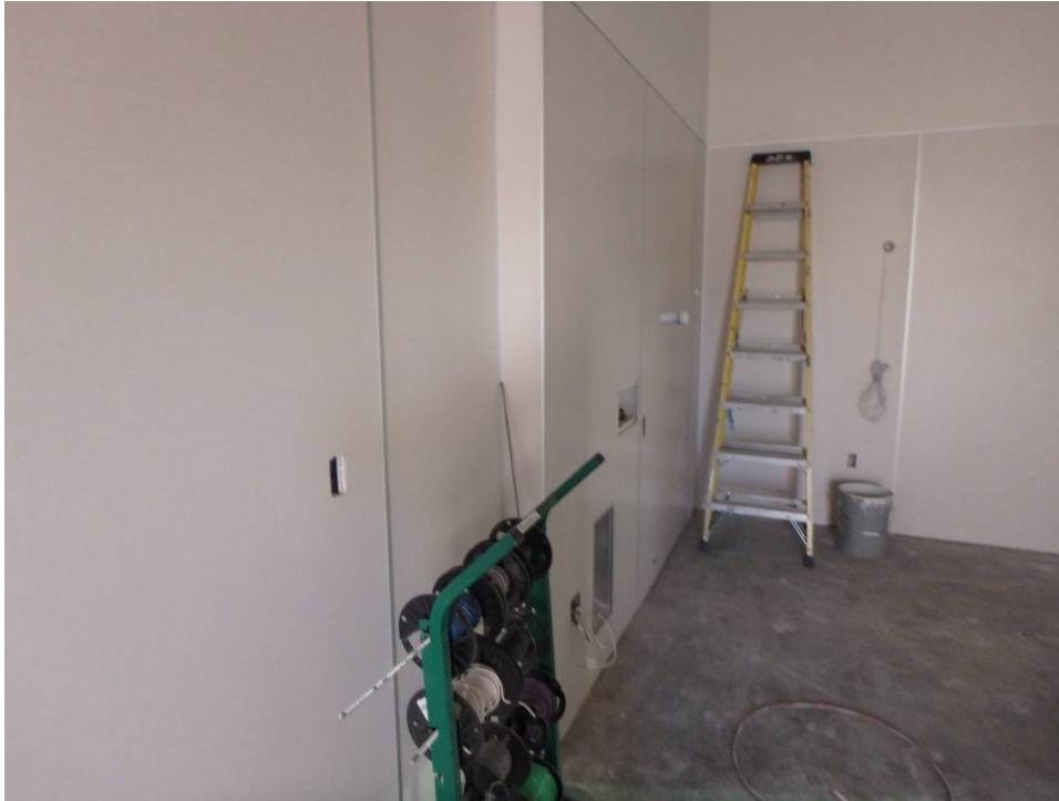
Kennel – northwest corner
