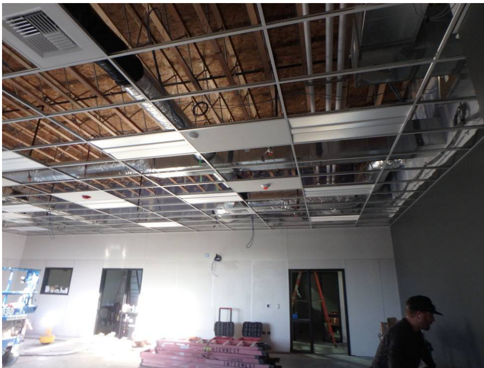
Looking at the west wall of the south classroom
