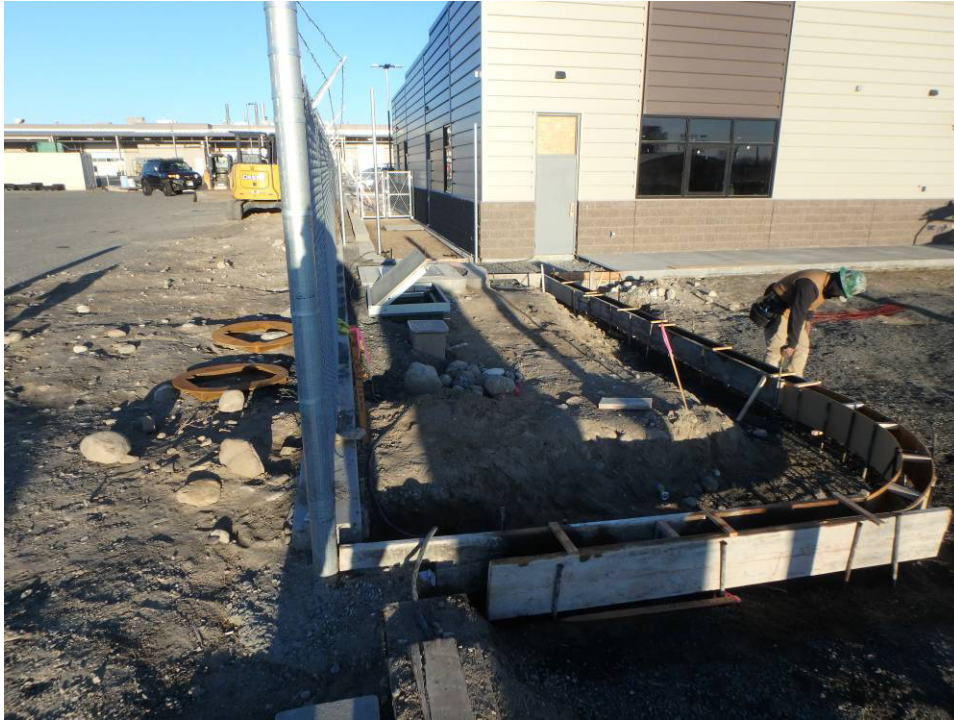
Southeast curb forms
