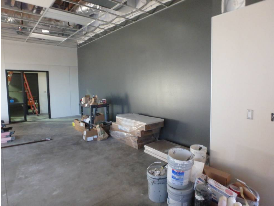
Looking at the north wall of the south classroom
