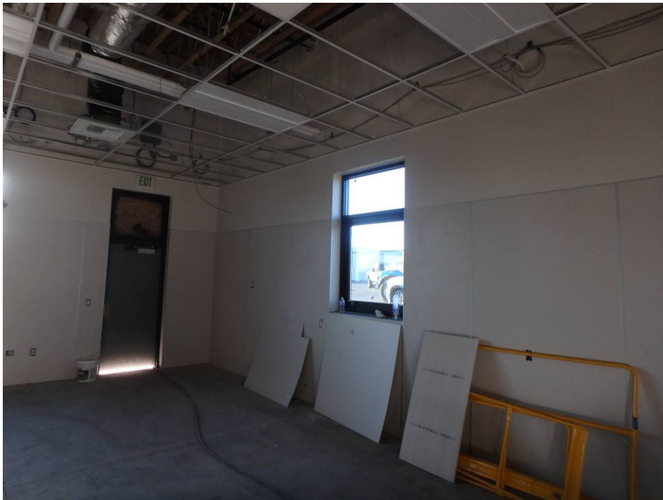
Looking at the southeast corner of the south classroom
