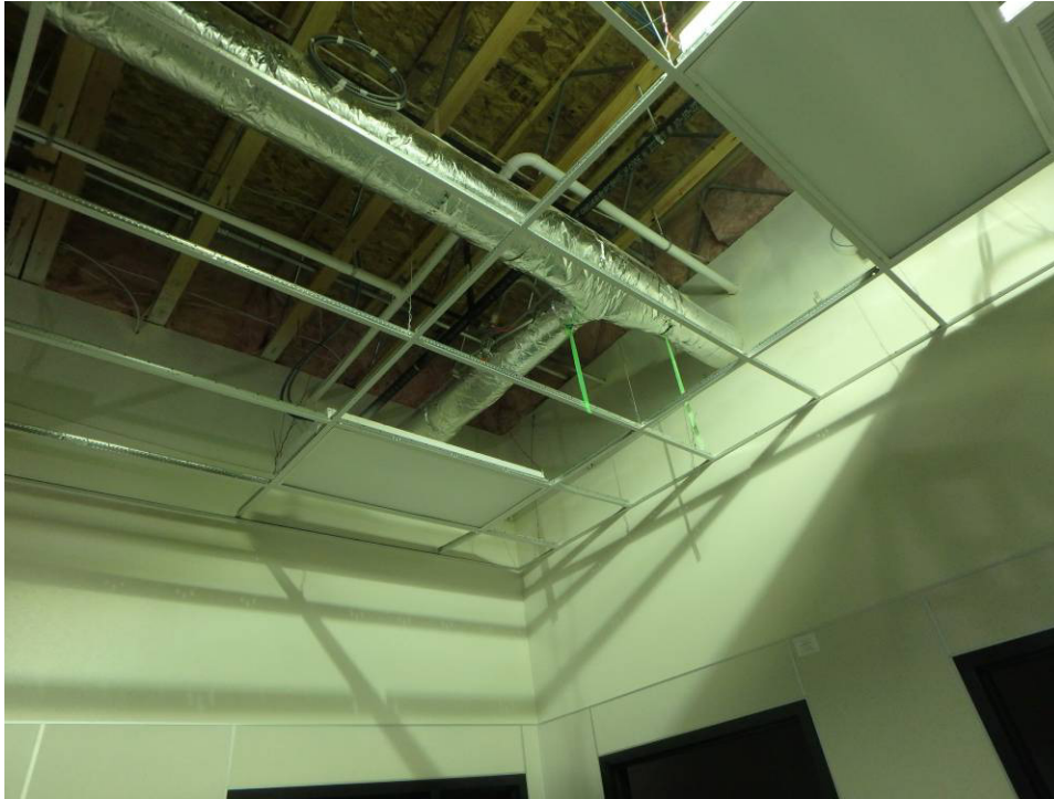
Lab northwest corner ceiling grid
