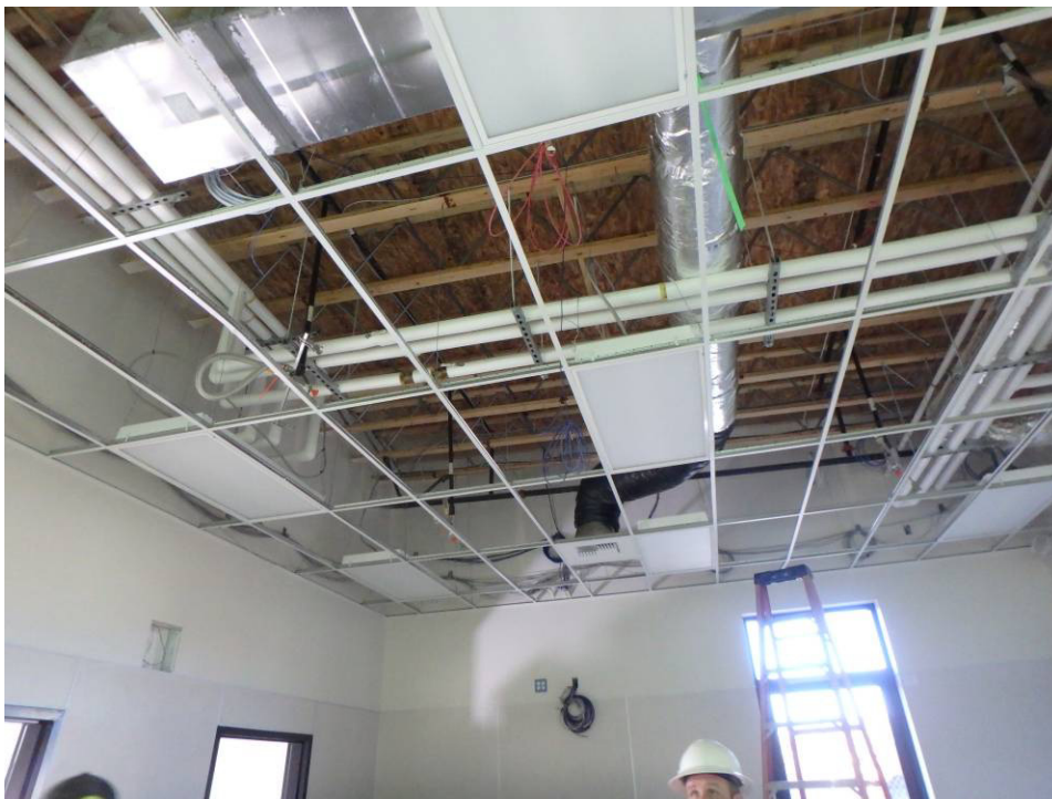
Ceiling grid in the lab – looking south
