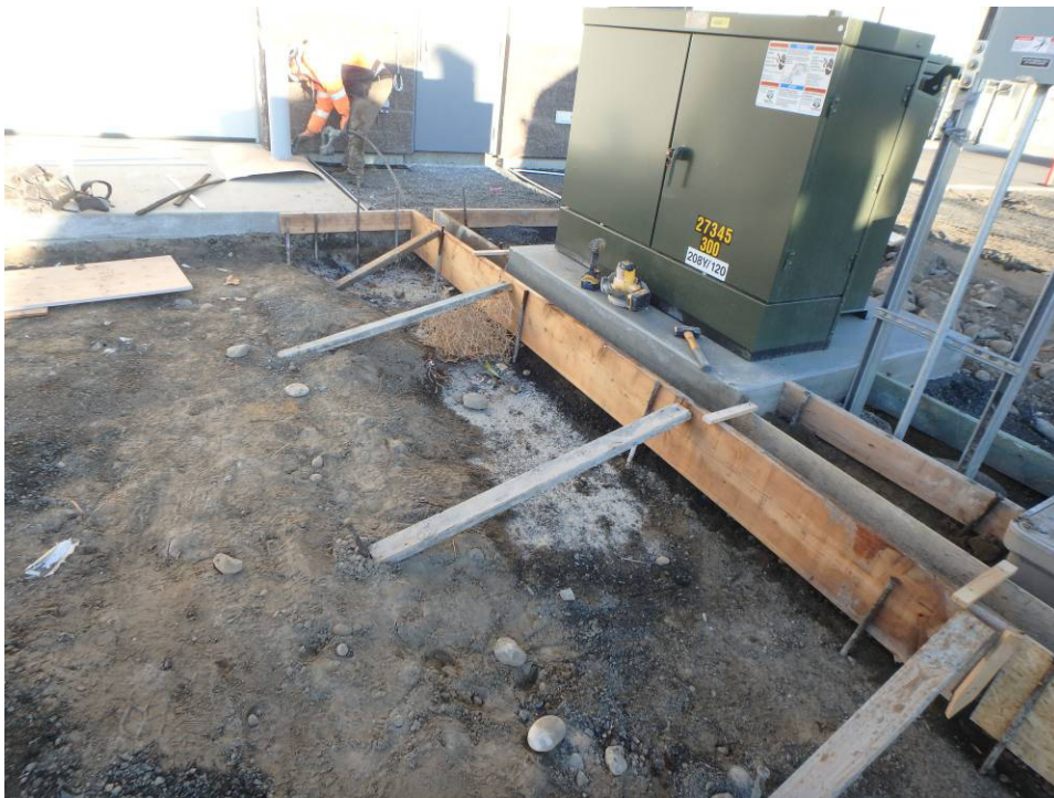
Curb formwork at transformer
