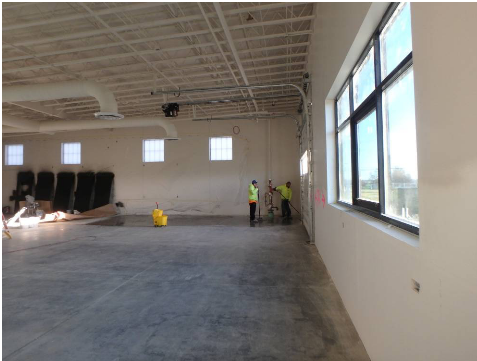
Looking north at the shop east wall, cleaning floors
