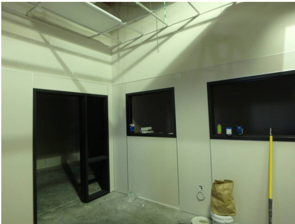
Lab northwest corner Exam room door
