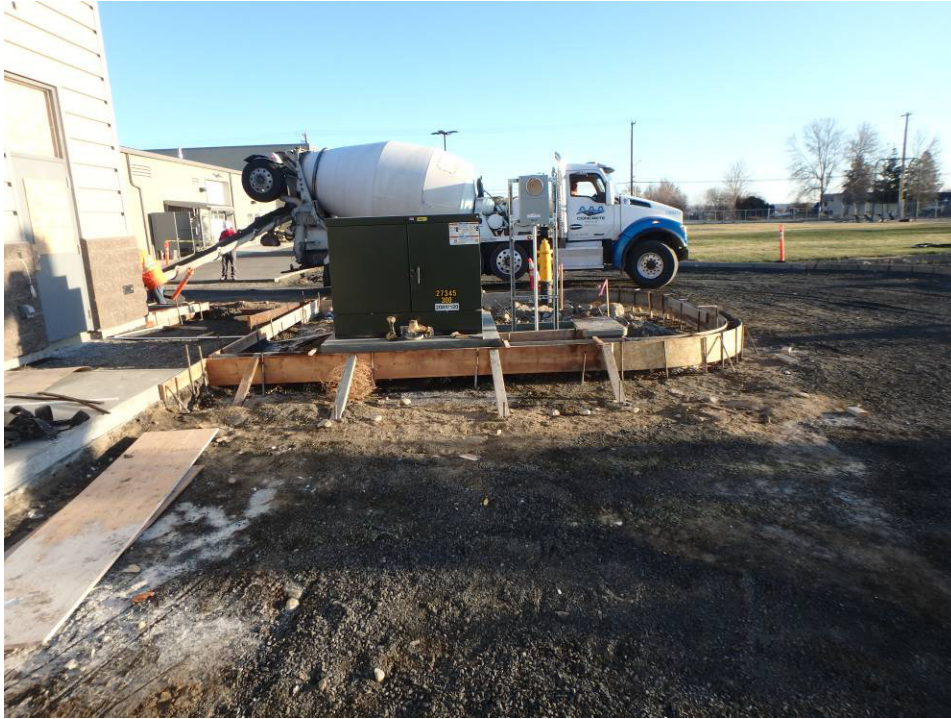
Northeast peninsula formwork
