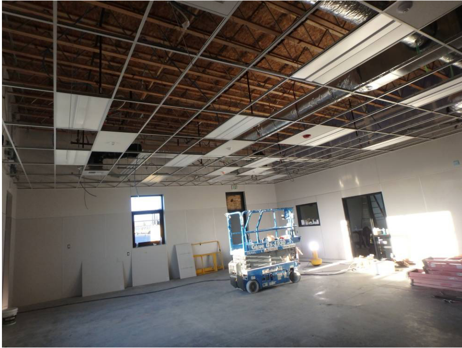
Looking at the southwest corner of the south classroom
