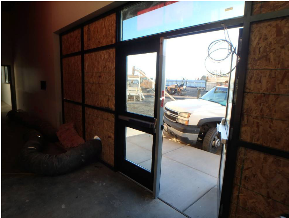
Main Entry doors
