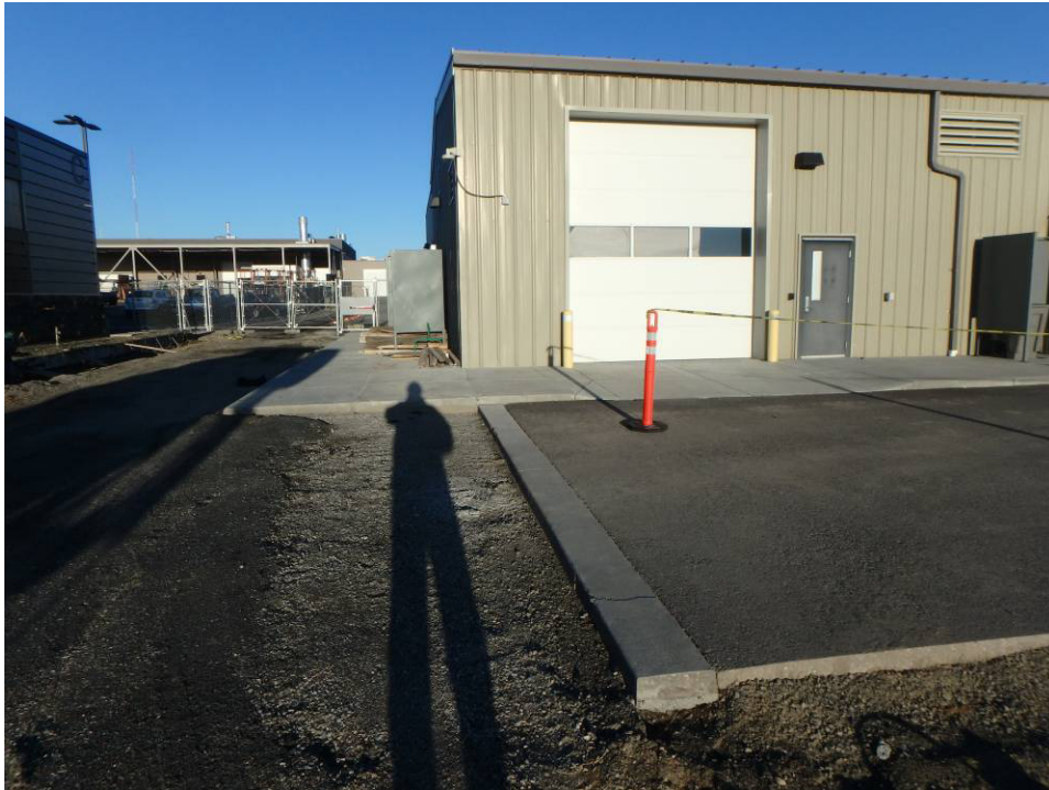
Looking west at the Tri Tech southeast curb
