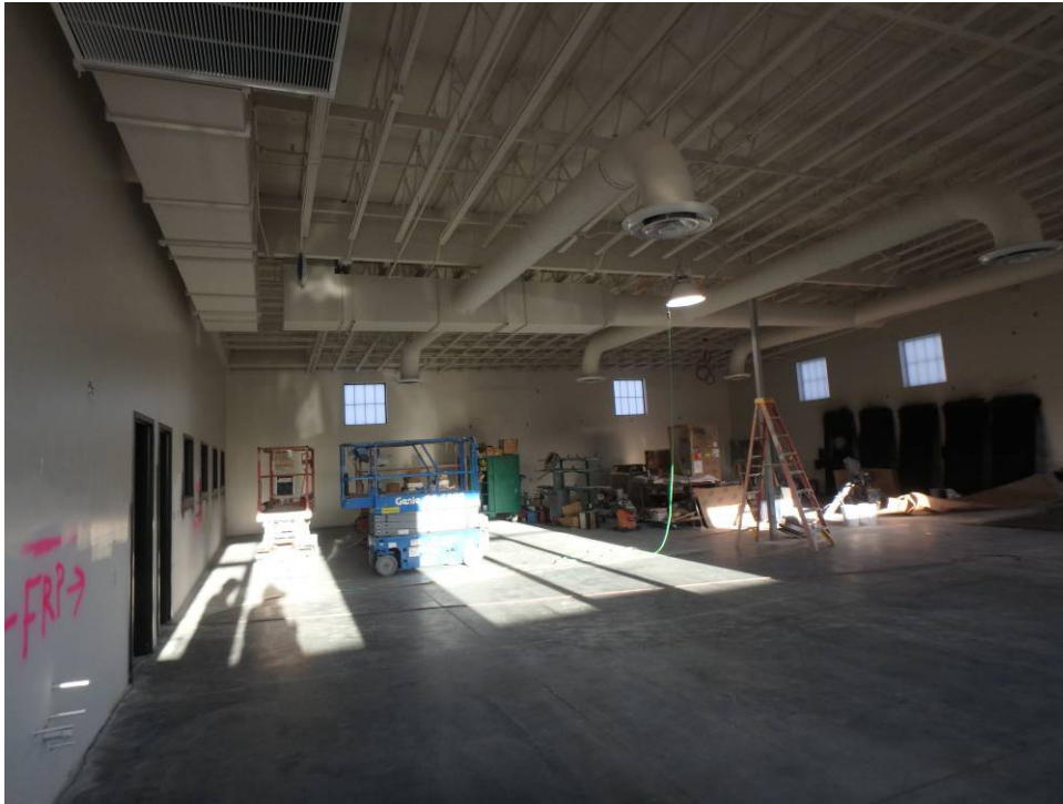
Looking west across the shop along the south wall
