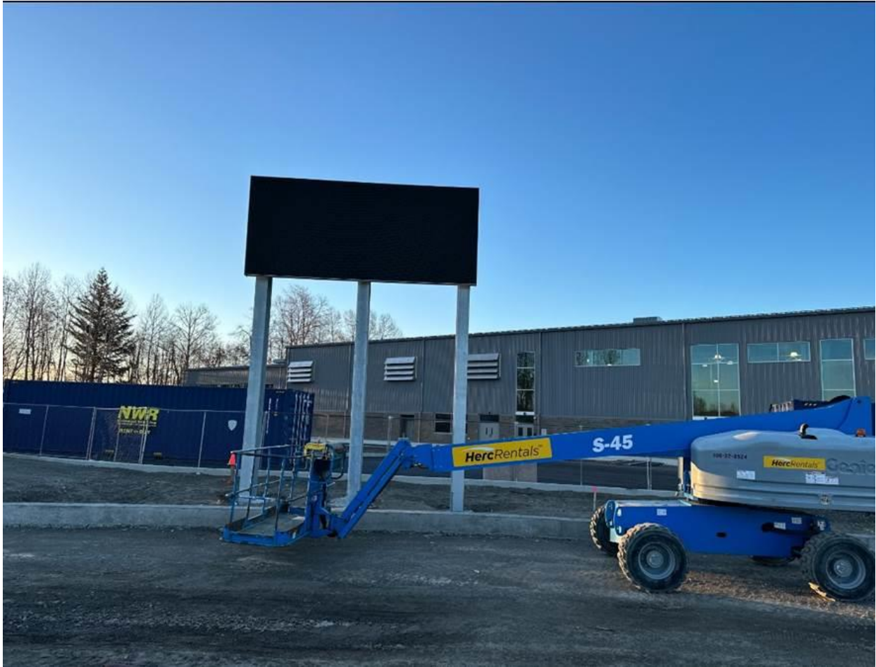
The football field's scoreboard is now installed
