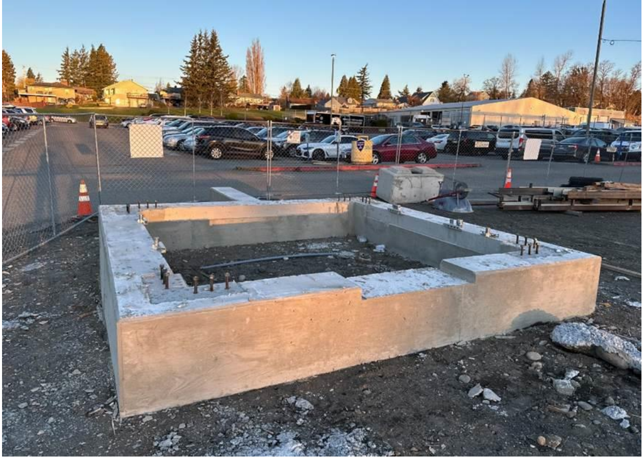
The foundation of the new football field's ticket booth
