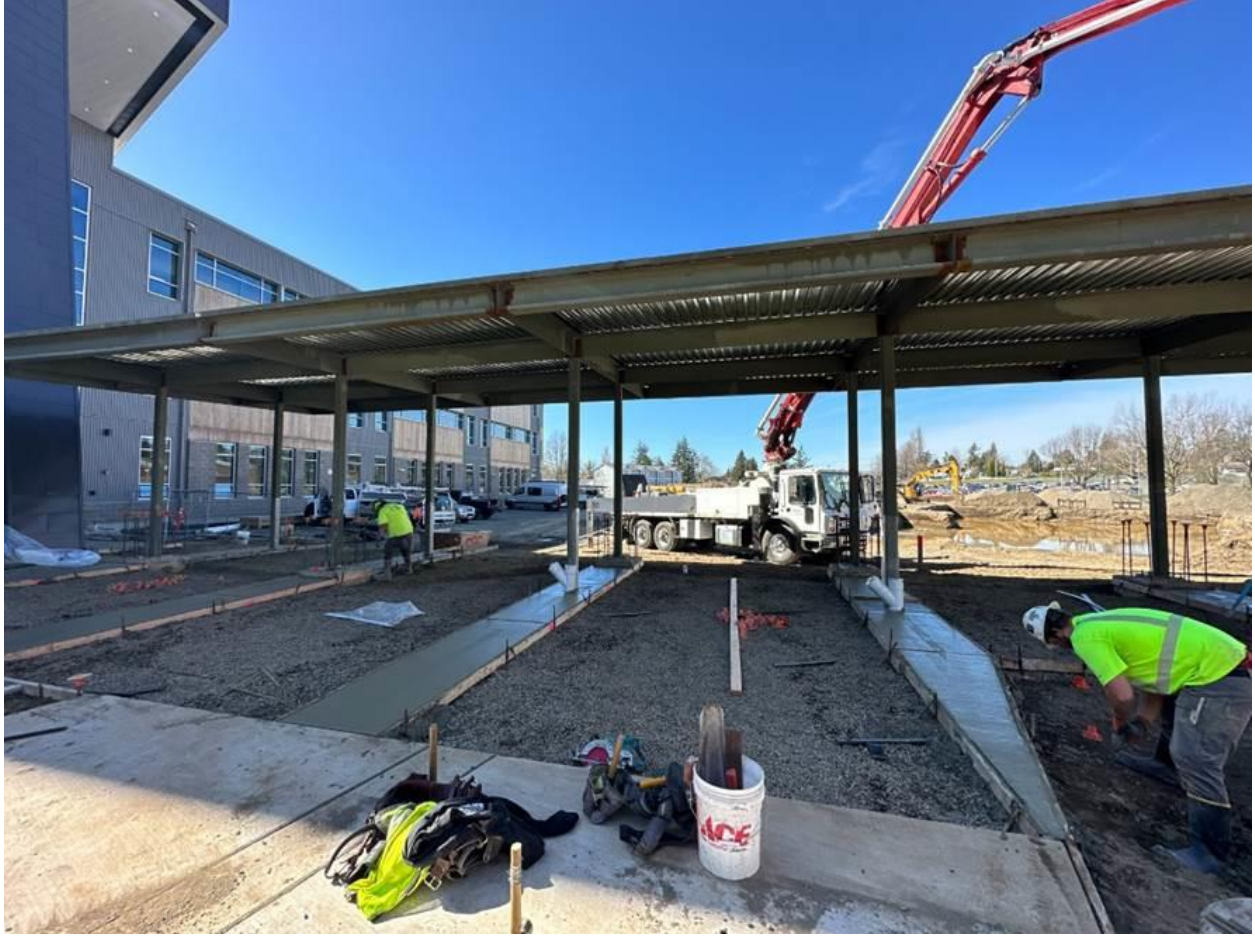
Concrete sidewalks being poured in the Commons' courtyard
