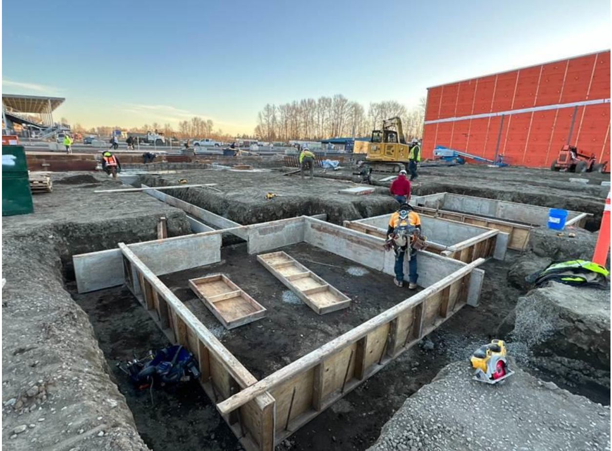
Foundation formwork in the CTE Wing area
