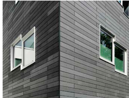
2 GLASS-FIBER REINFORCED CONCRETE SIDING AT SECOND FLOOR
