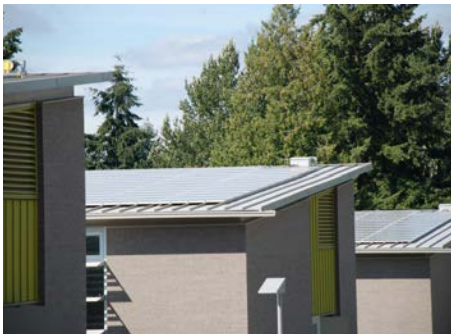
4 METAL STANDING SEAM WITH PHOTOVOLTAIC PANELS AND SKYLIGHTS ON UPPER ROOF
