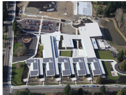
4 METAL STANDING SEAM WITH PHOTOVOLTAIC PANELS AND SKYLIGHTS ON UPPER ROOF
