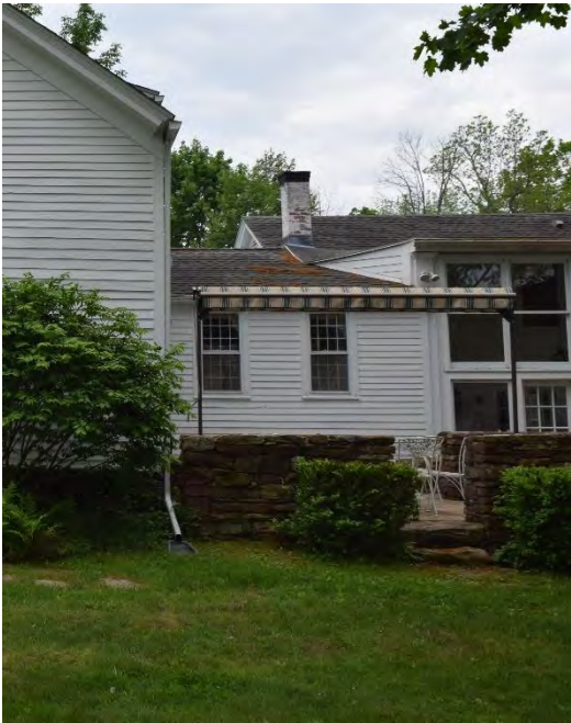
Nonfunctional chimney – cannot be seen easily from road
